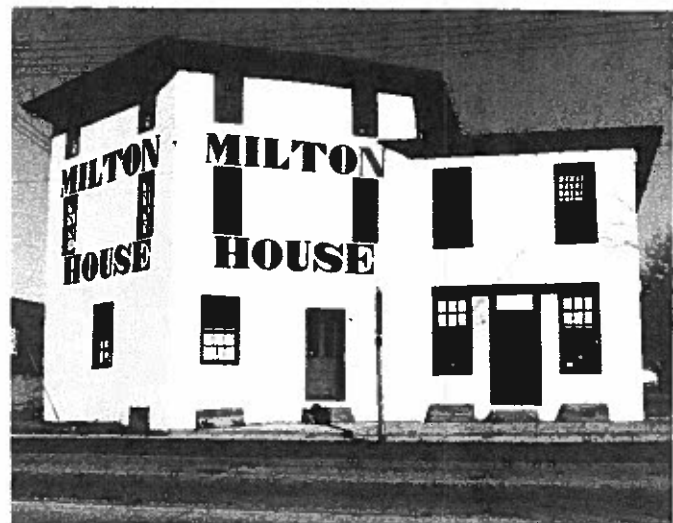
Fig. 1. Milton House, Milton, Wisconsin (1844). An early example of gravel wall construction with 12- to 15-inch thick monolithic concrete walls coated on the exterior with stucco. Photo: William B. Coney.
