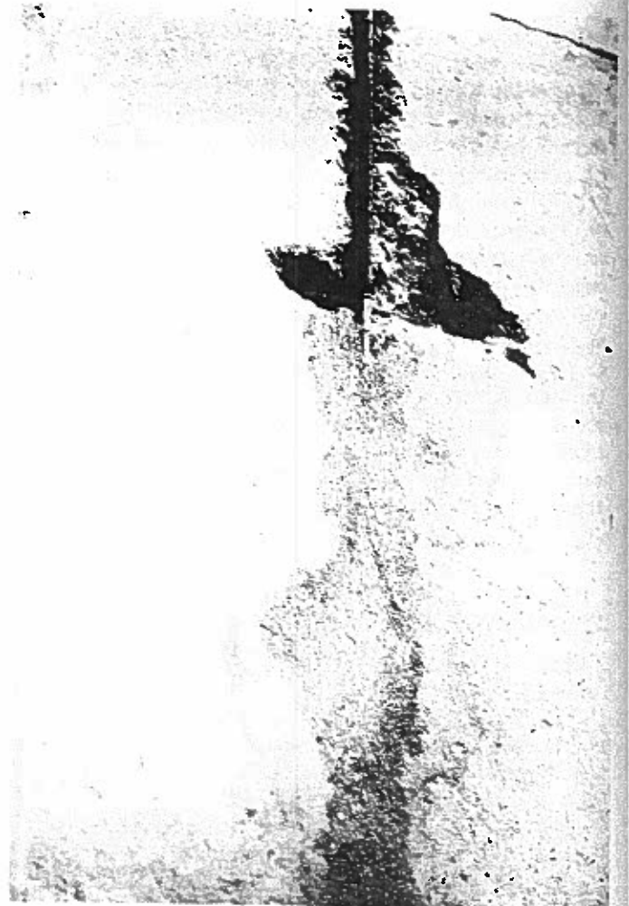
Fig. 12. Without proper preparation and correction of a pre-existing problem, repairs will fail. Insufficient concrete at the surface caused this patch around a reinforcing bar to fail within a year. In this case, a structural engineer should have assessed the need for this rod so close to the surface. Redundant rods are often cut out prior to patching. Photo: Alonzo White.
