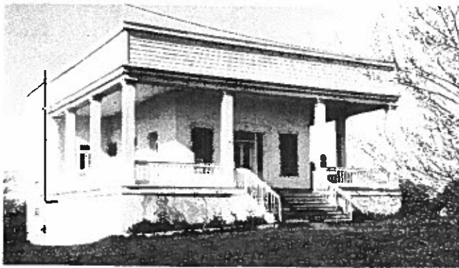
Fig. 2. Sebastopol House, Seguin, Texas (1856). This Greek Revival dwelling is one of the few remaining poured-in-place concrete structures in this Texas town noted for its construction of over 90 concrete buildings in the mid-nineteenth century. The high parapets surrounding the flat roof were lined and served as a water reservoir to cool the house. Photo: Texas Historical Commission.
