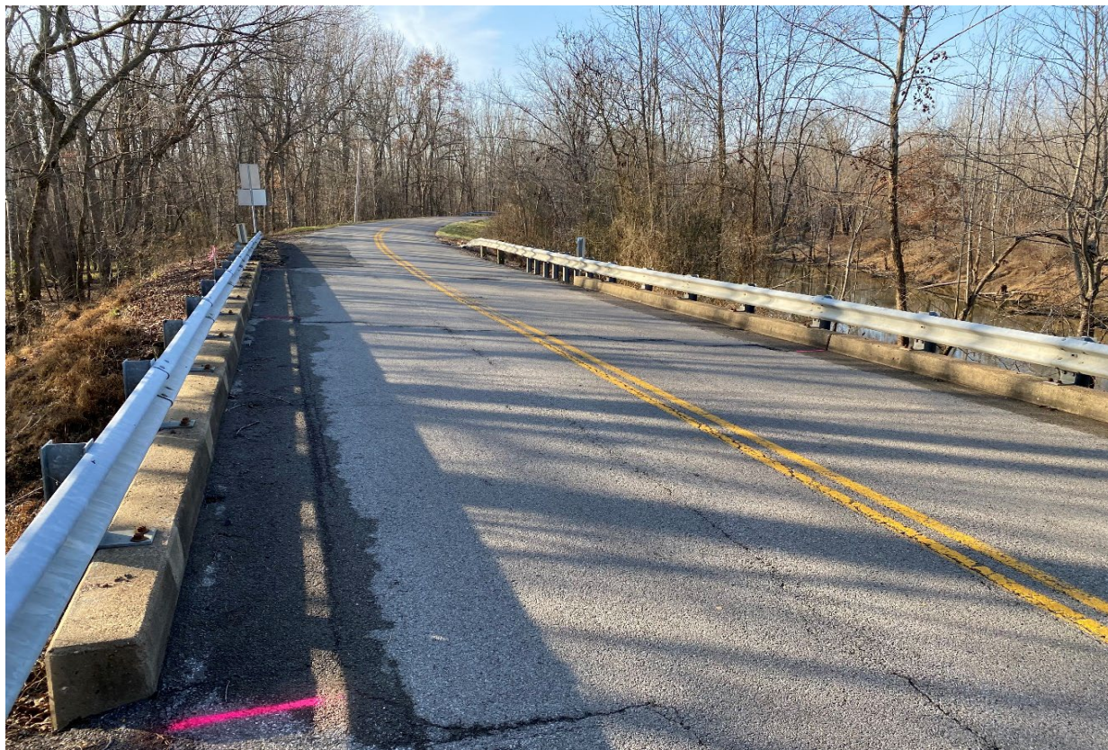
I - IMG_2693 Bridge Surface - Facing W.JPG
