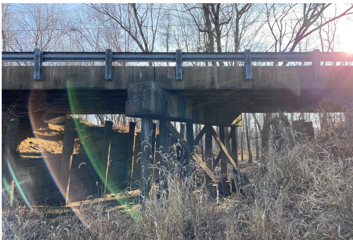
2 - IMG_2694 Bridge Below Deck - Facing S.JPG
