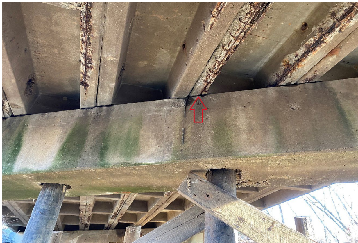
5 - IMG_2697 Joint at Pier Cap - Facing E - Sample I-10108-3.JPG
