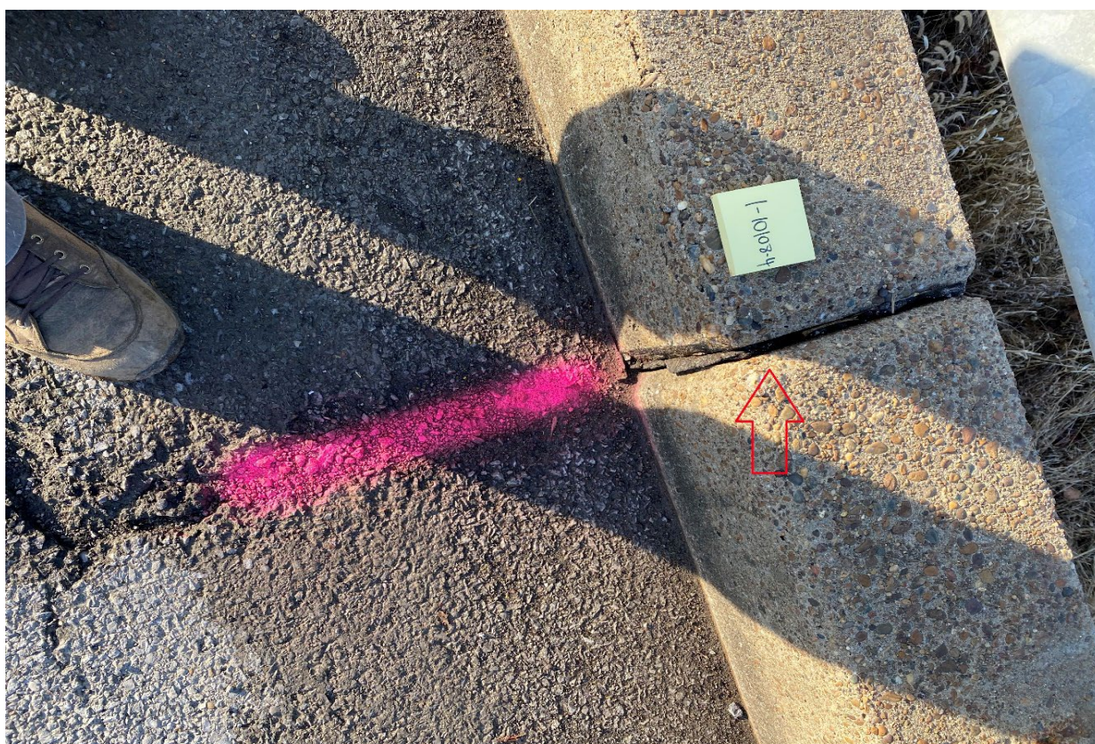
6 - IMG_2698 Joint in Curb and Road - Facing N - Sample I-10108-4.JPG
