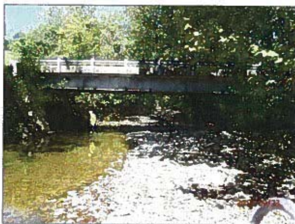
LOOKING UPSTREAM AT BRIDGE
