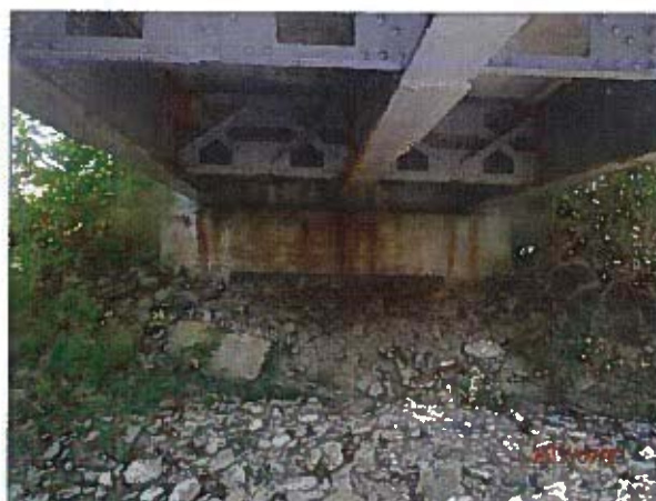
VIEW OF ABUTMENT #2
