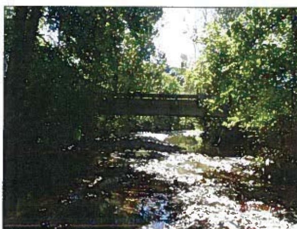
LOOKING DOWNSTREAM AT BRIDGE
