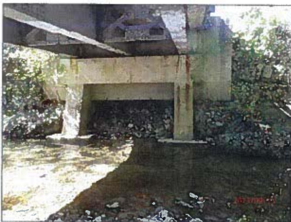
VIEW OF ABUTMENT #1
