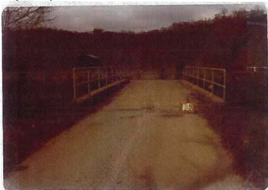
1980s photo of bridge showing original pipe railing
