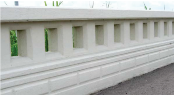
Figure 70: C412 Rail – Traffic Face
