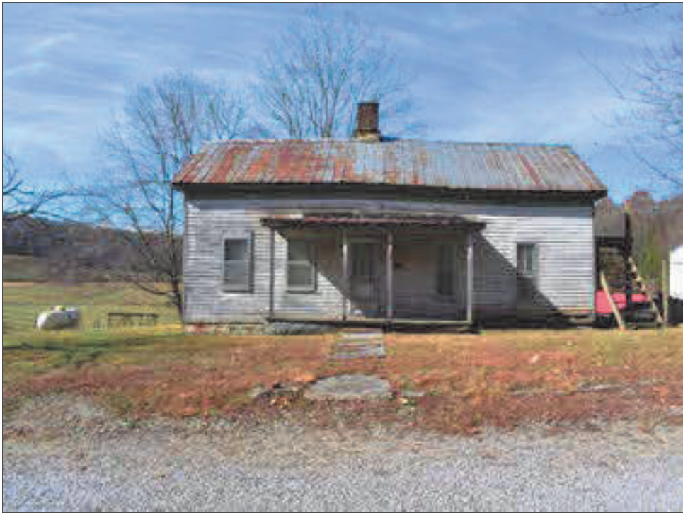
Photo 1: East elevation of Field Site 1.
