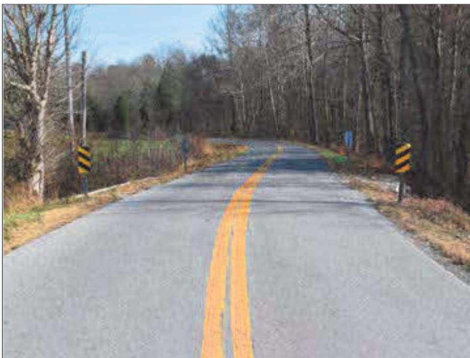
Photo 1: Facing east toward Bridge No. 016B00031N.
