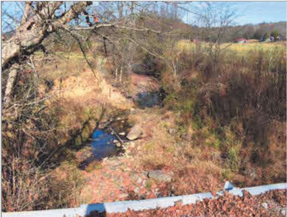
Photo 4: Facing north from Bridge No. 016B00031N.
