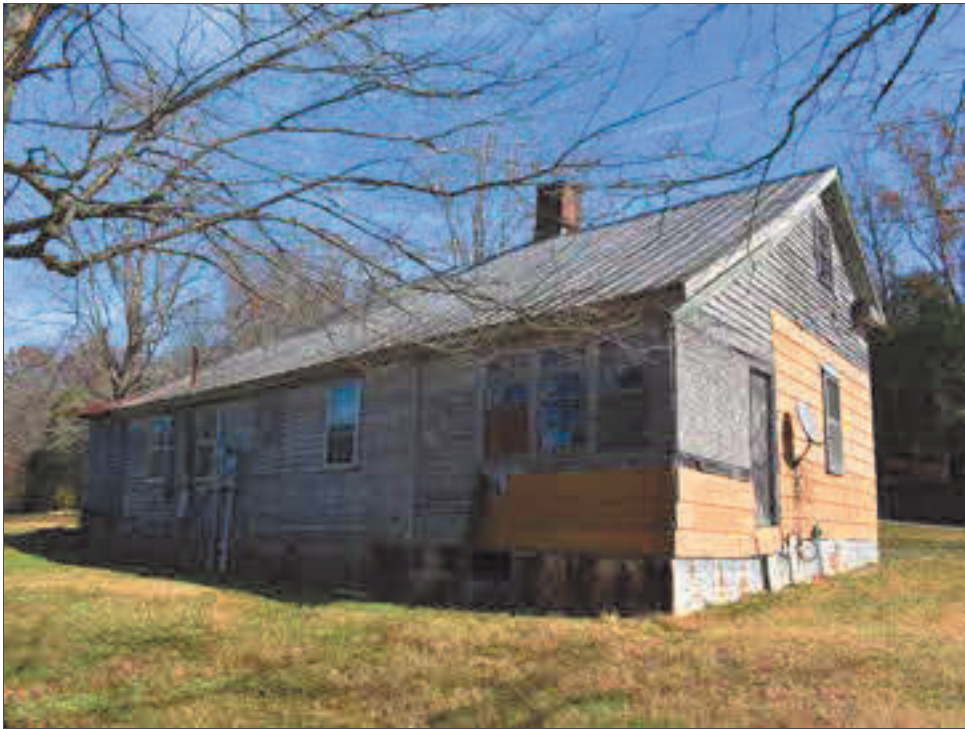
Photo 3: South and west elevations of Field Site 1.
