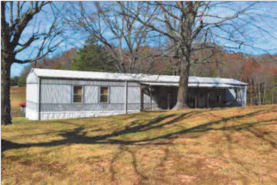
Photo 9: South and east elevations of mobile home.
