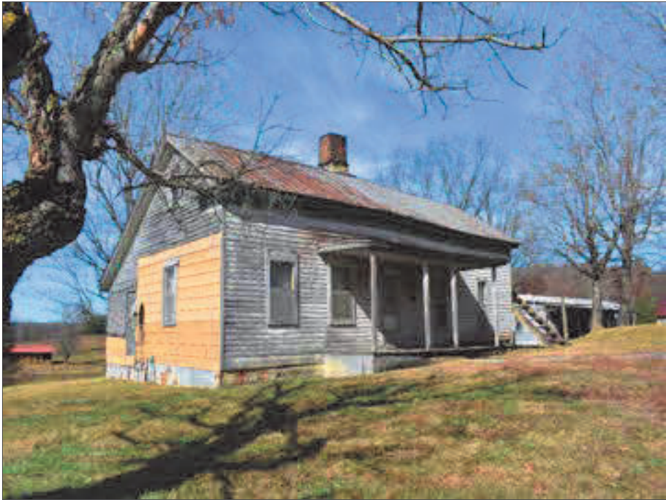
Photo 2: South and east elevations of Field Site 1.
