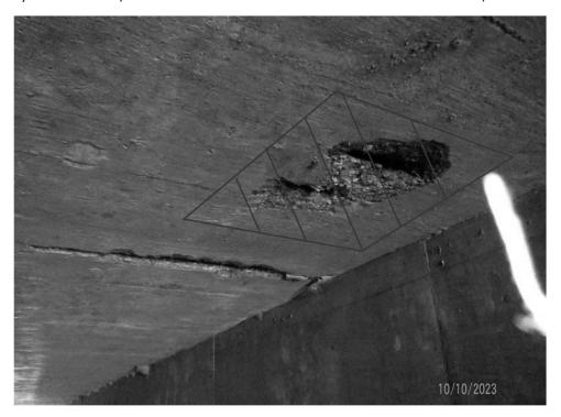
2) PATCH SPALL WITH EXPOSED REBAR IN SIDEWALL AT WEEPHOLE, 5 SF CONCRETE PATCHING:
