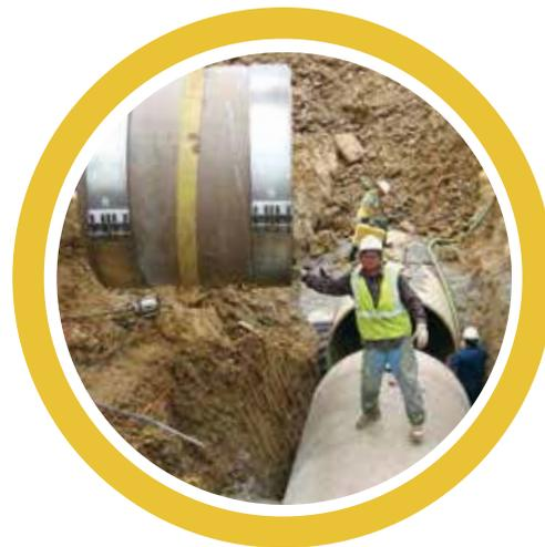
**Note:** When using mechanical joints, torque bolts to the minimum needed for sealing - maximum 25 ft-lbs.
