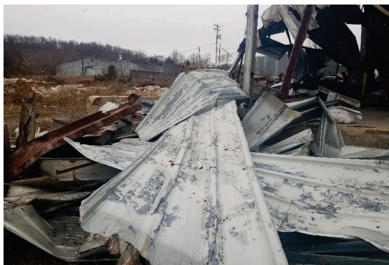
Demolished metal wall with peeling coating
