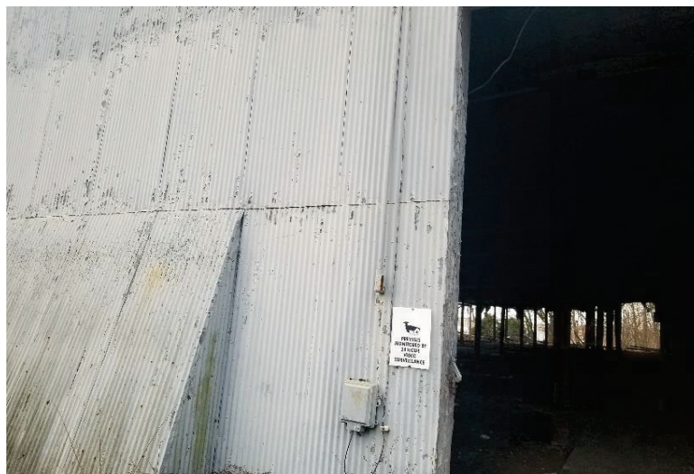
Back Building Exterior wall with peeling coating
