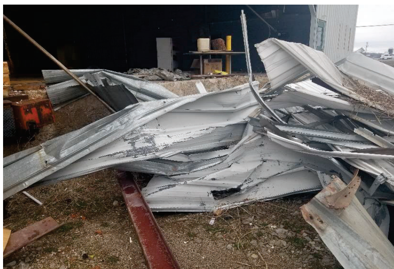
Demolished siding and roofing with peeling coating
