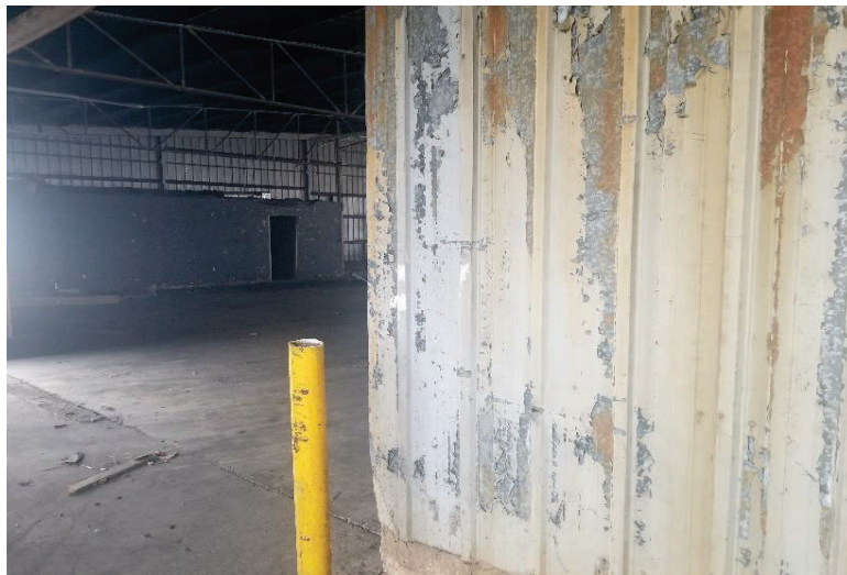
Front Building Interior metal wall with peeling coating
