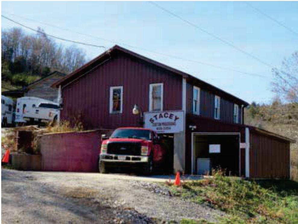
Commercial building (resource C), looking west.
