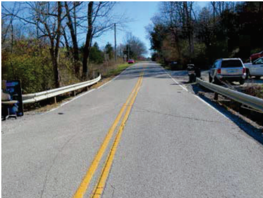
Bridge deck and railings, looking southeast.
