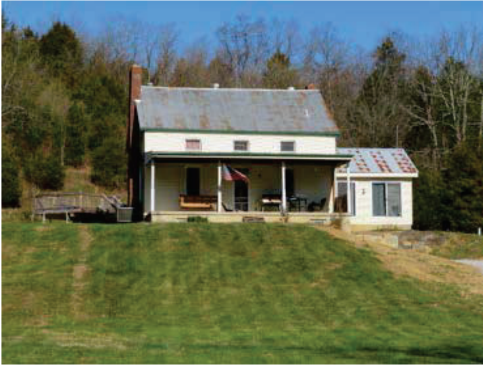
Façade of residence, looking north.
