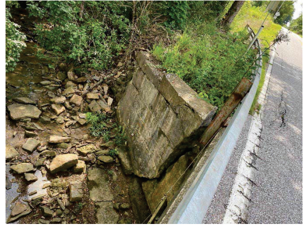
Bridge abutment and streambed.
