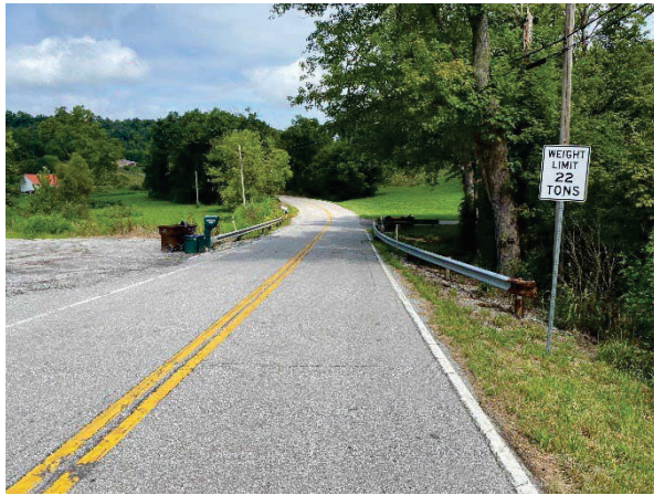
View of bridge from roadway
