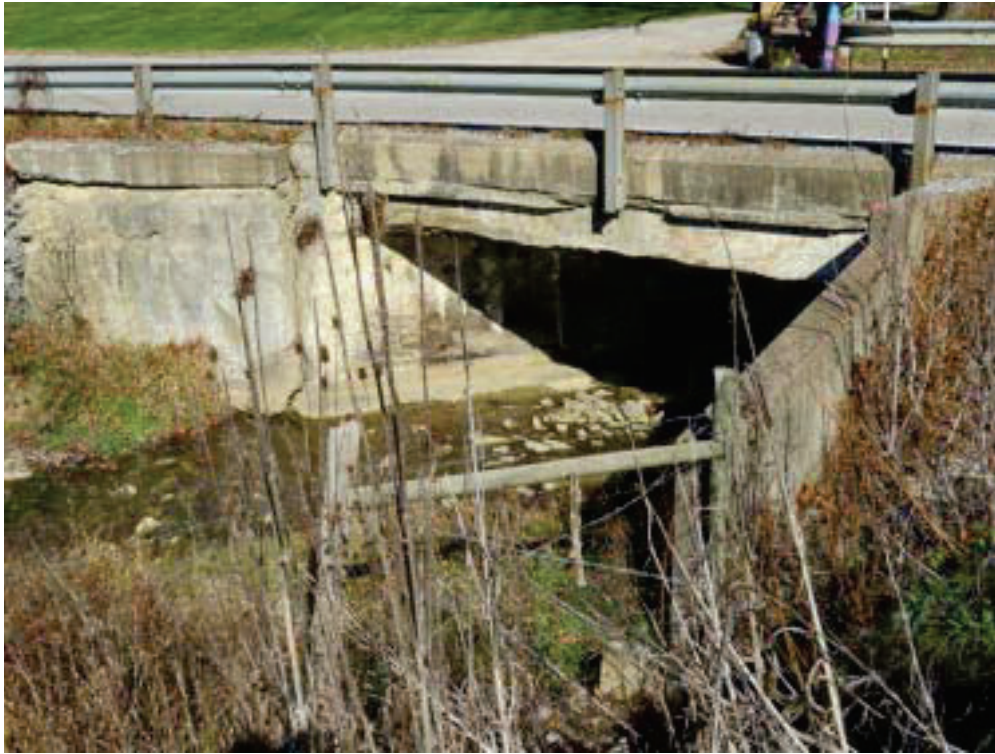
Side view of bridge, looking north.
