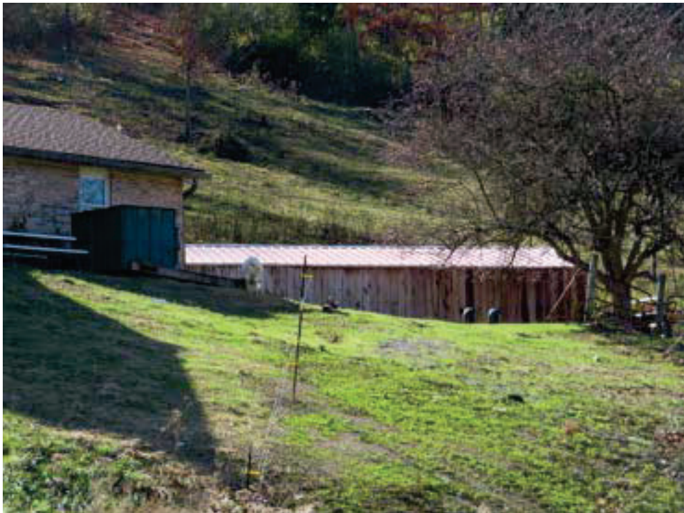
Outbuilding (Resource D), looking southwest.
