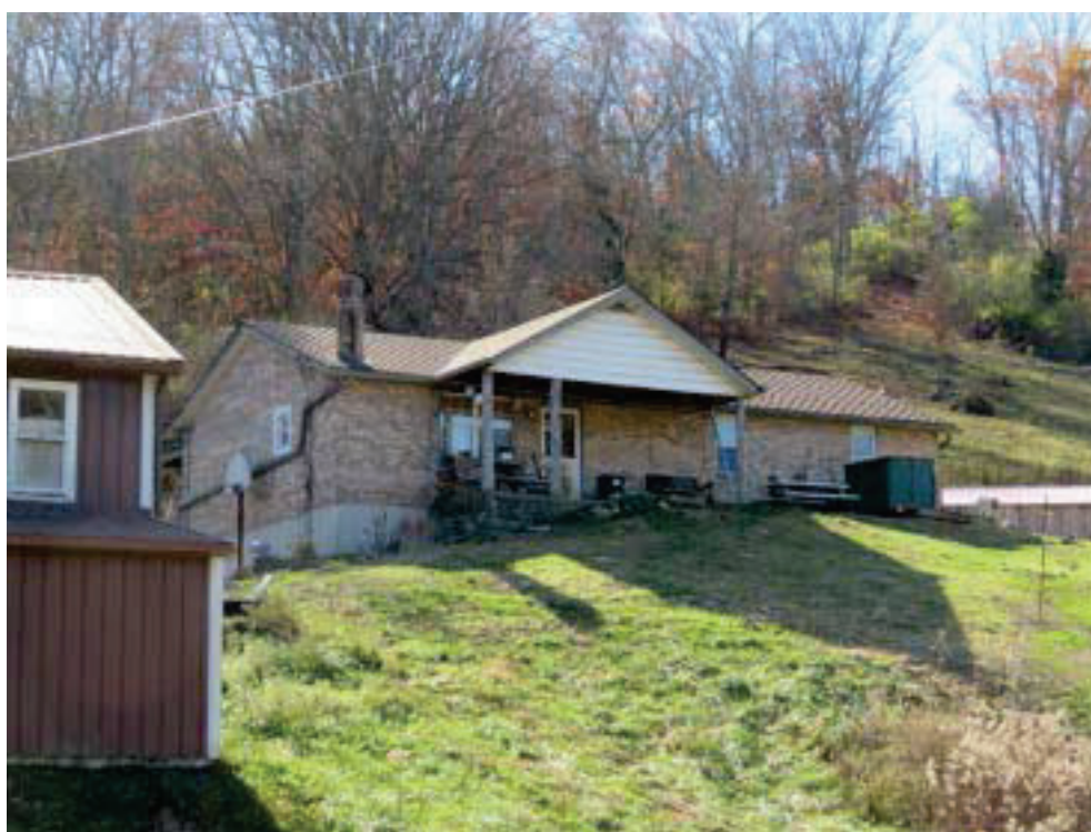
Façade and east elevation of residence, looking southwest.
