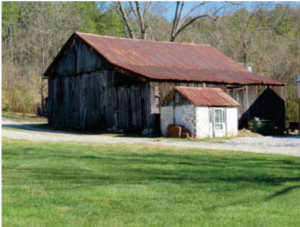
Barn (Resource C) and outbuilding (Resource D), looking northeast.
