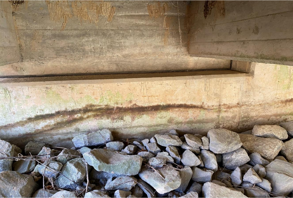
3 - IMG_2627 Joint in Abutment - Facing E.JPG
