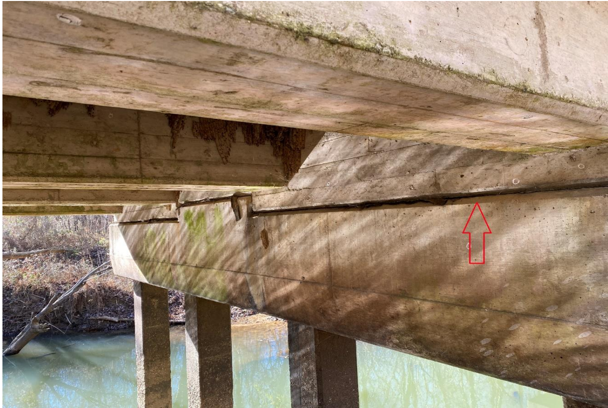
7 - IMG_2629 Horizontal Joint Above Pier - Facing W - Sample I-10102-4.jpg
