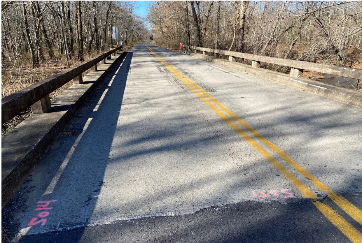
1 - IMG_2624 Bridge Surface - Facing W.JPG
