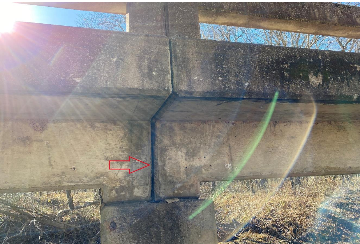
6 - IMG_2628 Vertical Joint Above Pier - Facing S - Sample I-10102-3.jpg
