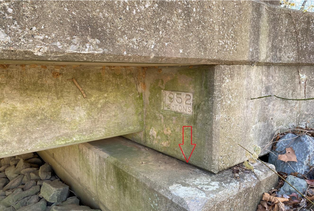
5 - IMG_2623 Joint in Abutment - Facing W - Sample I-10102-2.jpg
