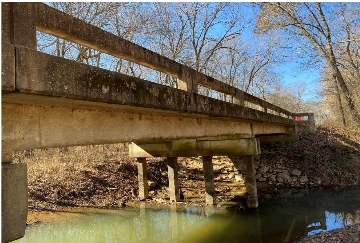
2 - IMG_2630 Bridge Below Deck - Facing W.JPG
