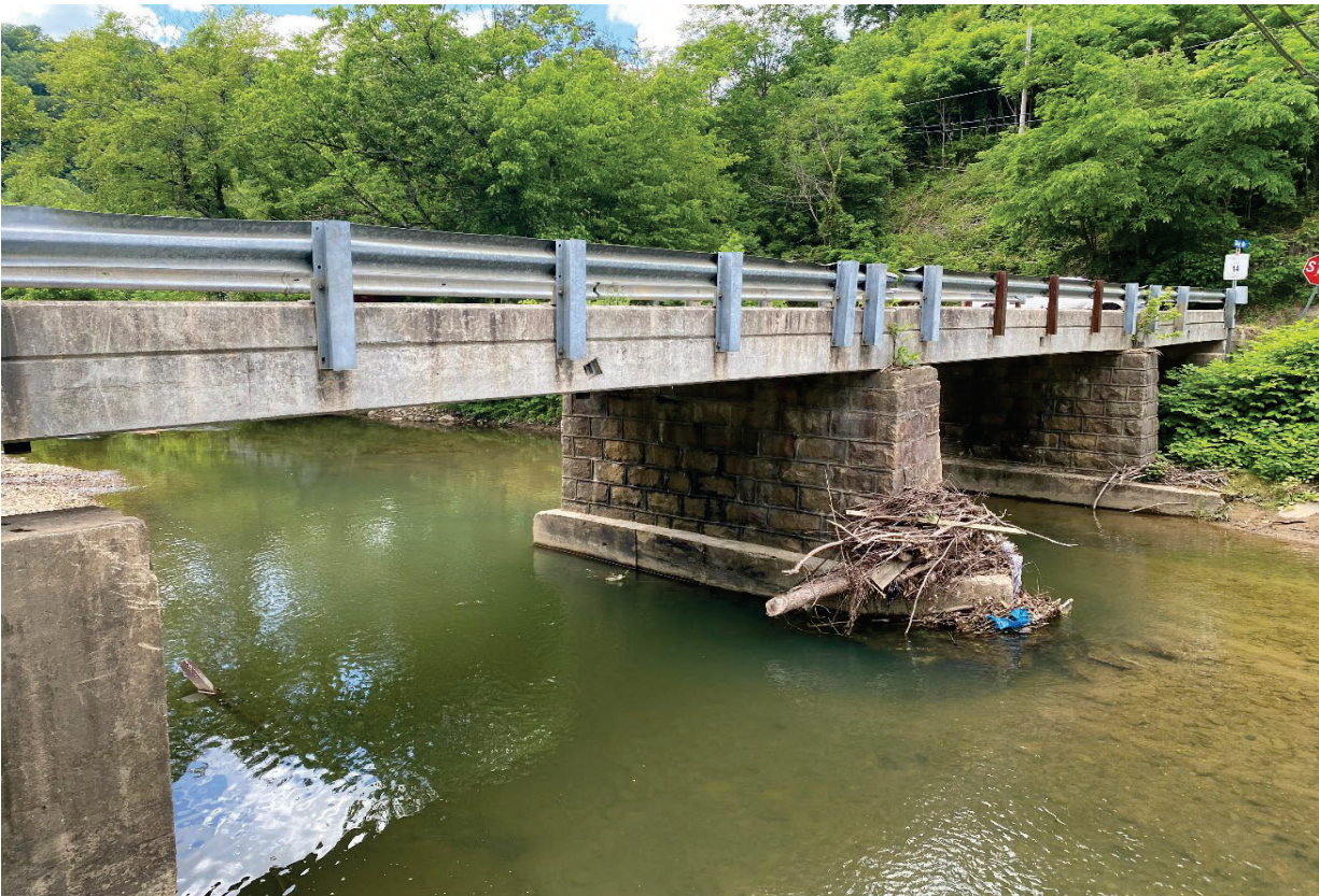
2 - IMG_3238 Bridge Below Deck - Facing W.JPG
