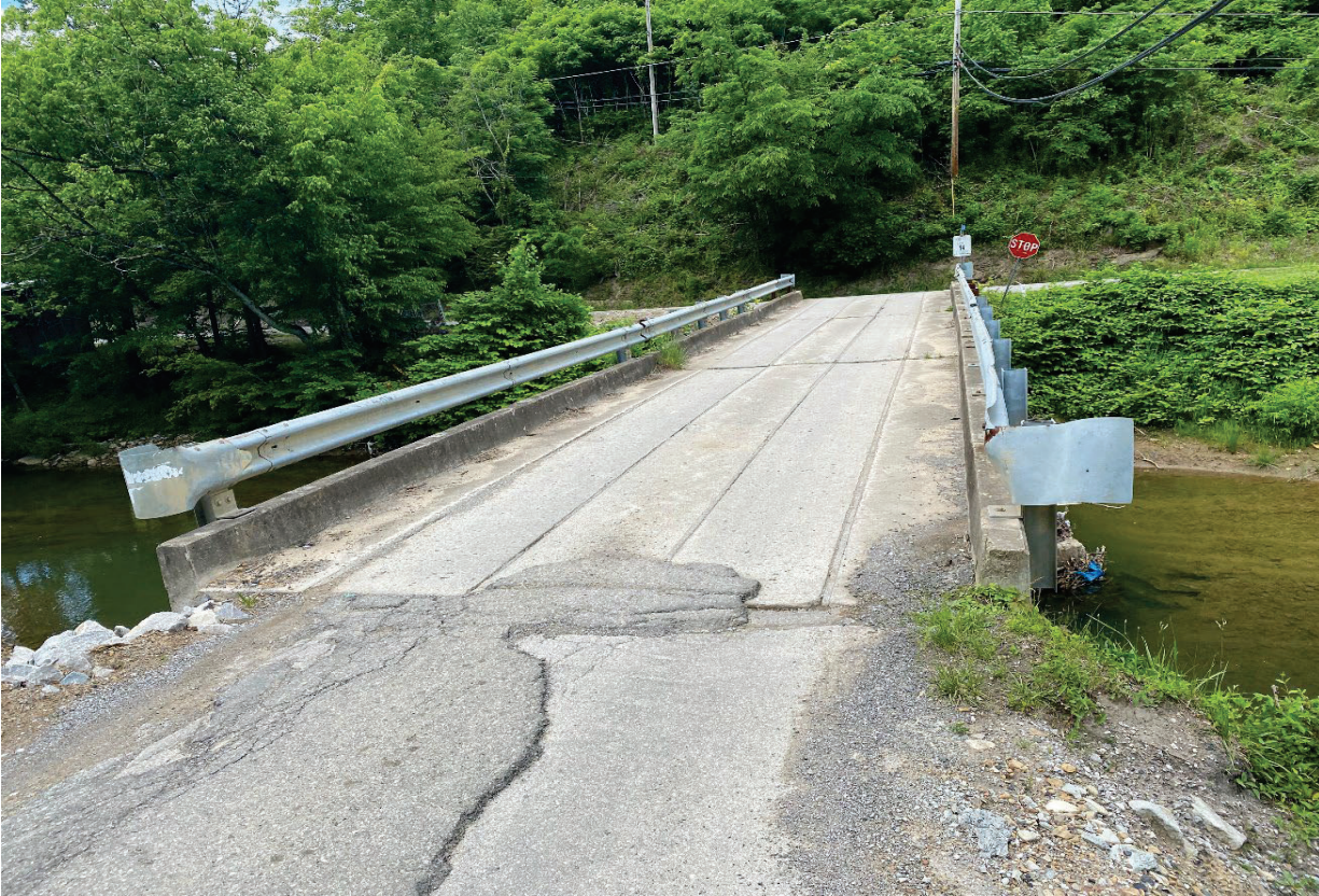
1 - IMG_3239 Bridge Surface - Facing W.JPG
