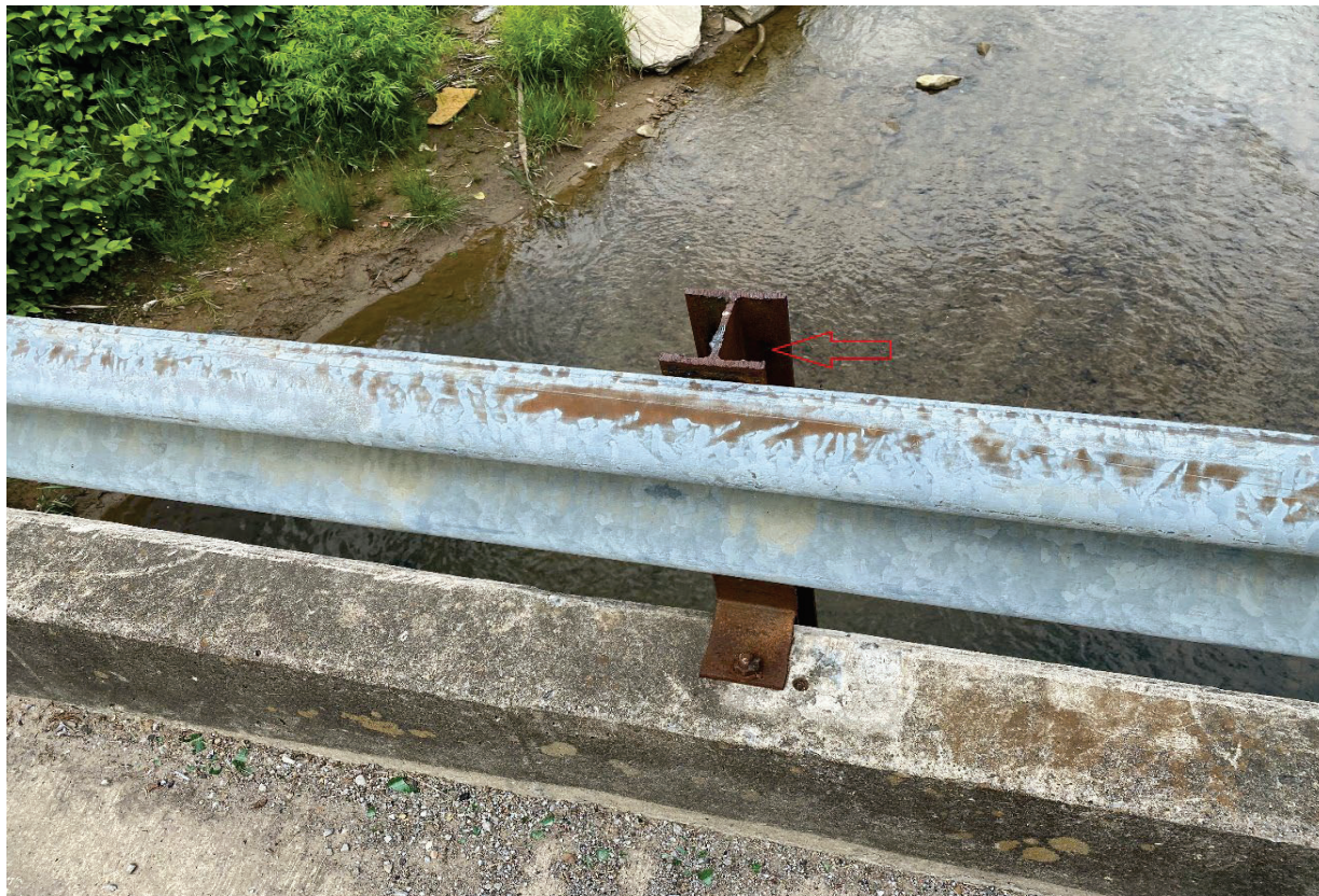
3 - IMG_3241 Metal Guardrail Support - Facing N - Sample 12-10145-1.jpg
