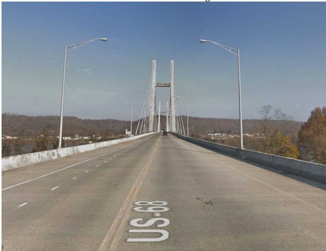
Bridge looking east
