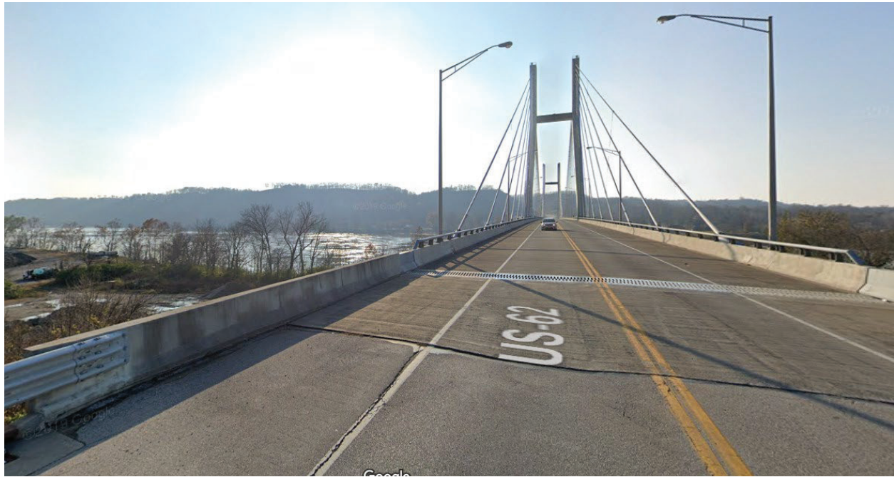
Bridge looking west
