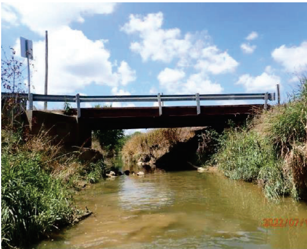
Downstream Elevation, looking West
