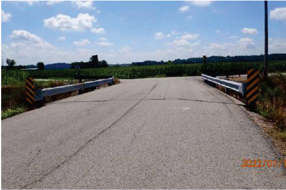
North Approach, looking South
