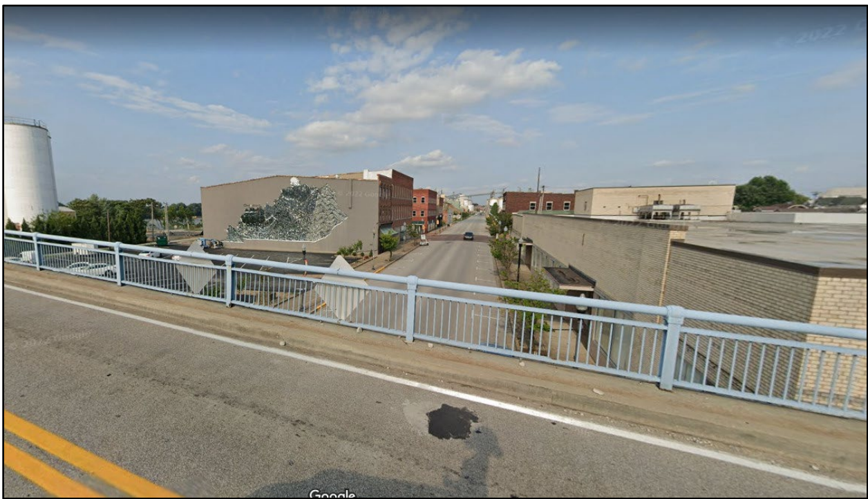
Looking northeast from bridge approaches
