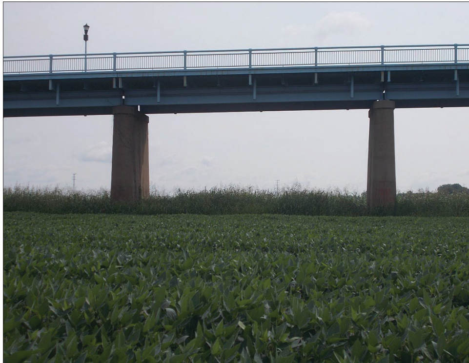
Photo 3: Glover Cary Bridge over the Ohio River, Indiana side; August 8, 2023
