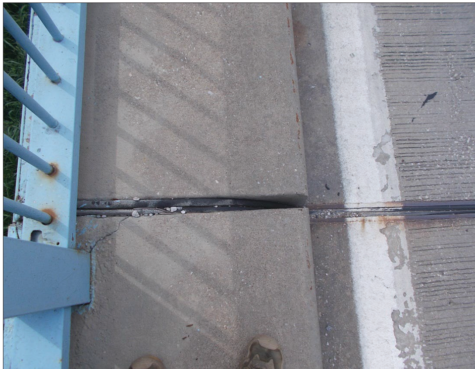
Photo 7: Example of potential bat roosting habitat if not filled with expansion joint, there were no exposed crevices like this; August 8, 2023
