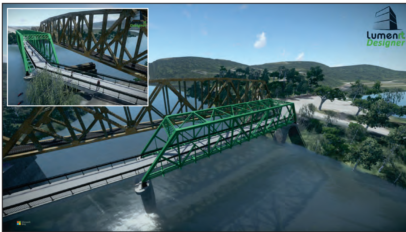
Figure 7. Alternative 4b – Rehabilitation of Main Truss with New Approaches and Substructure Shifted Slightly Downstream
