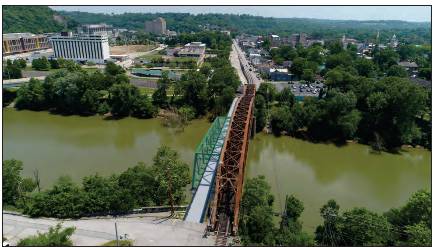
Figure 4. Alternative 2 - Complete Rehabilitation
