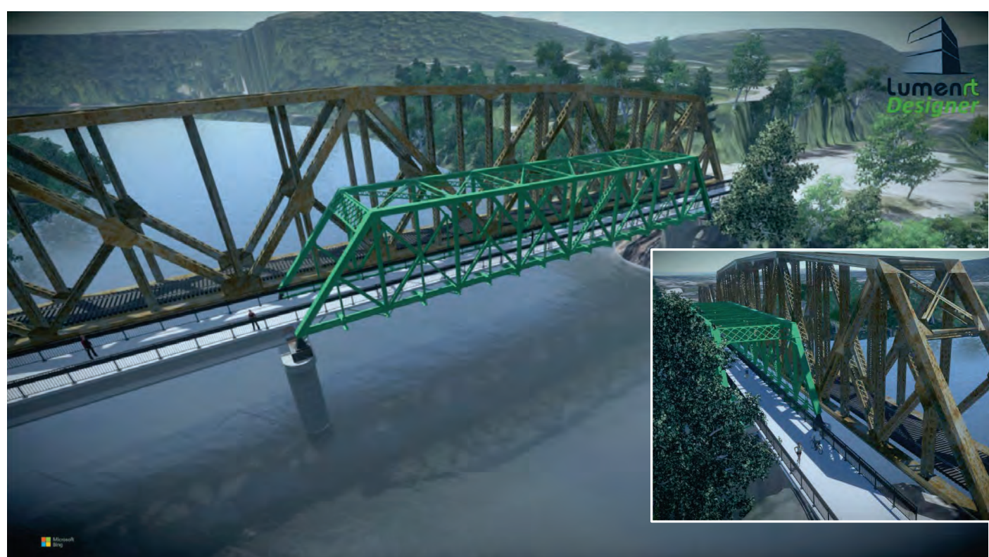
Figure 6. Alternative 4a – Rehabilitation of Main Truss with New Approaches on Existing Alignment
