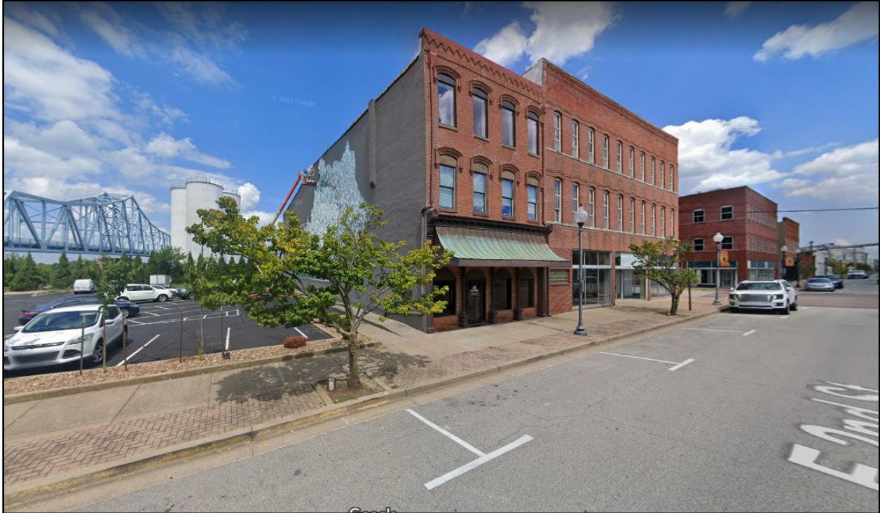
Looking north at second street
