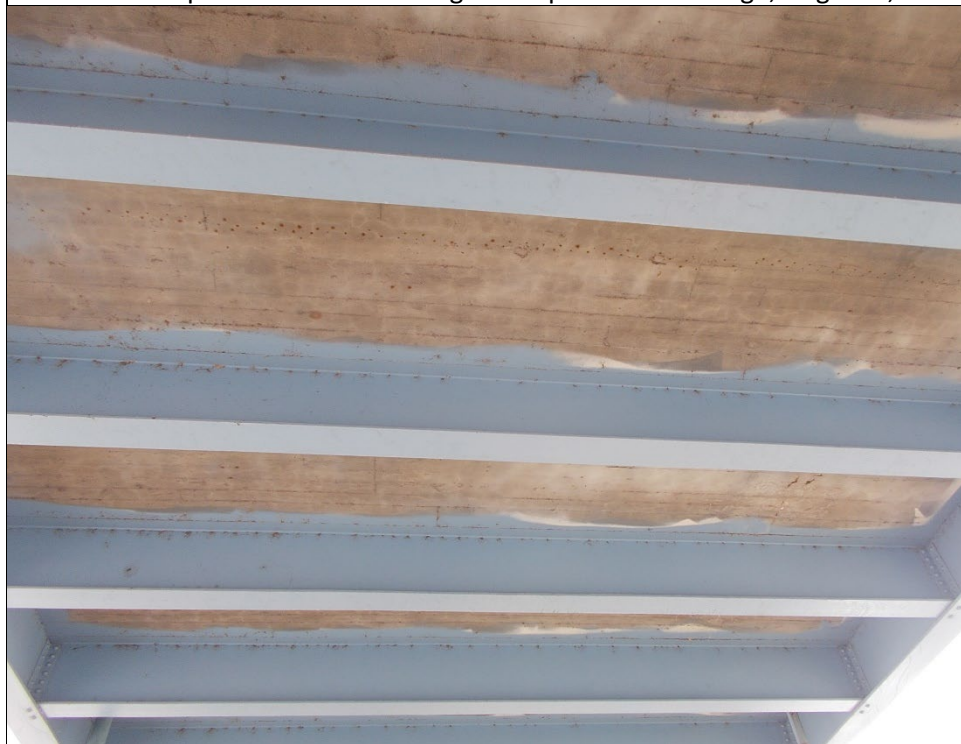
Photo 6: Example of the concrete decking under parts of the bridge; August 8, 2023
