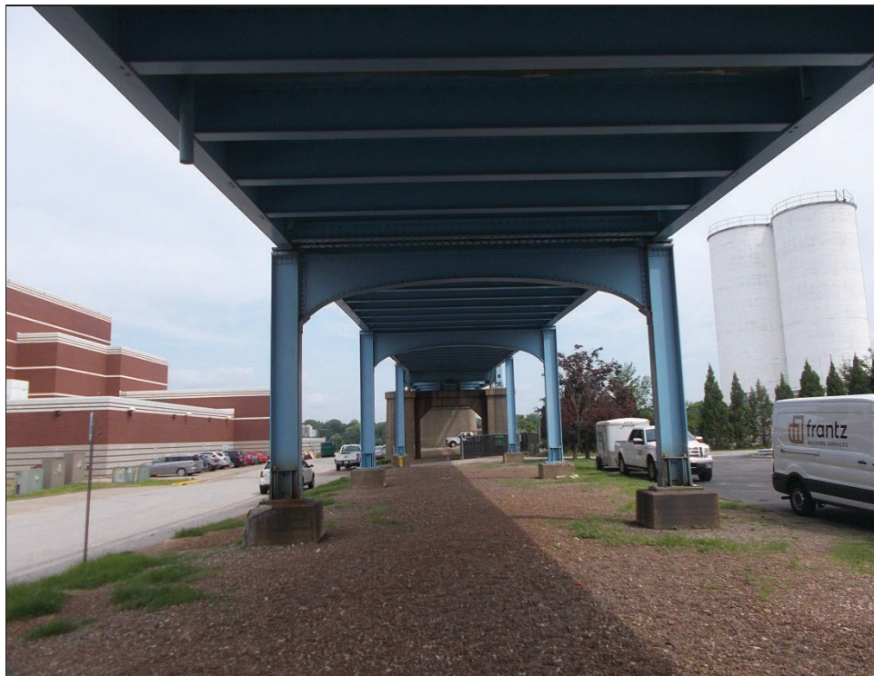
Photo 4: Glover Cary Bridge over the Ohio River, Kentucky side; August 8, 2023
