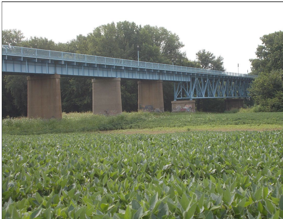
Photo 2: Glover Cary Bridge over the Ohio River, Indiana side; August 8, 2023
