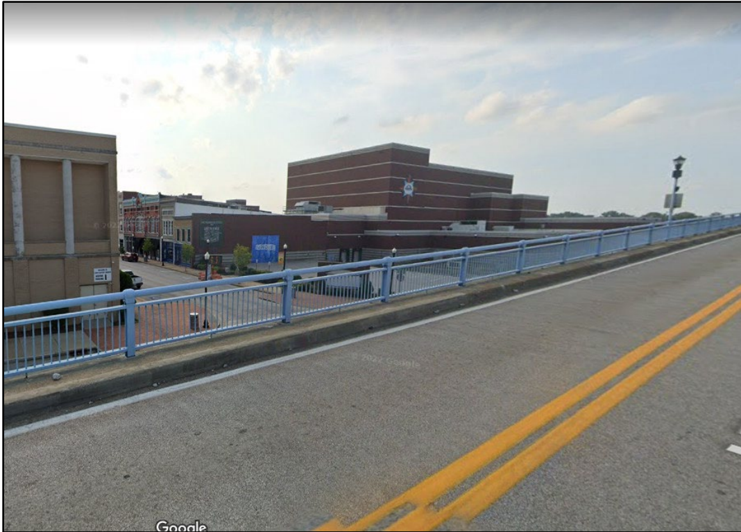
Looking northwest from bridge approaches
