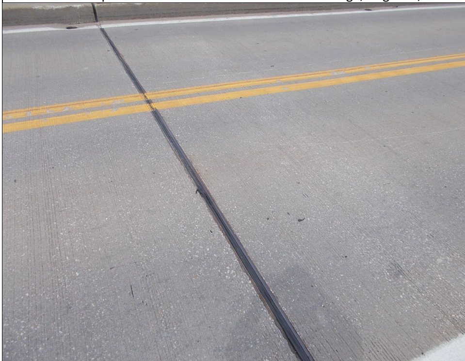
Photo 8: Example of the one-inch rubber compression expansion joint; August 8, 2023
