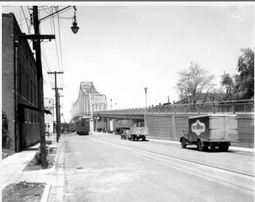
Glover Cary Bridge (also known as the Blue Bridge) in Owensboro, Kentucky, 1941. Source: UASC, Thomas Mueller collection, MSS 247-1476.
