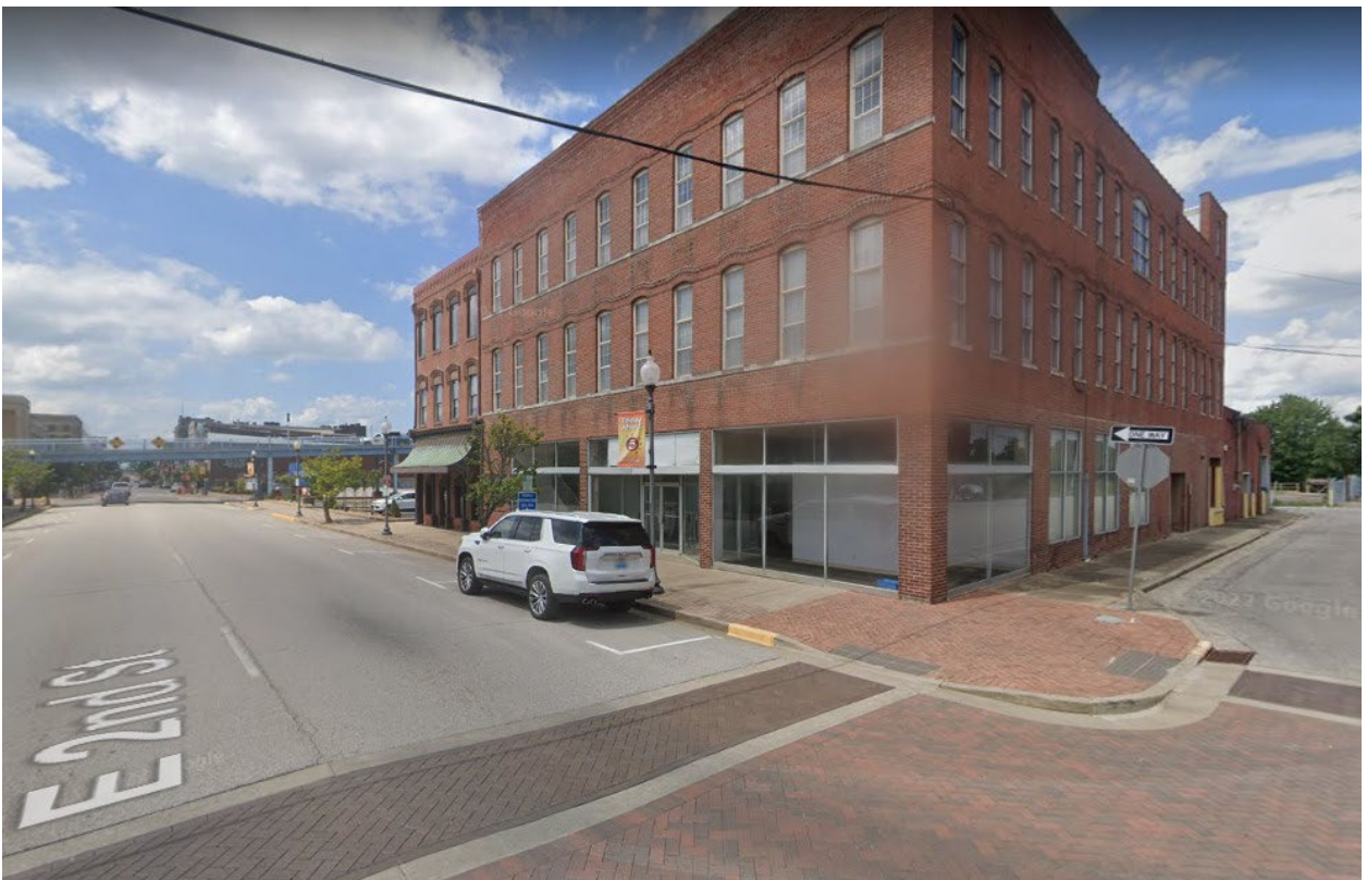
Intersection of 2 nd street and Crittenden looking west
