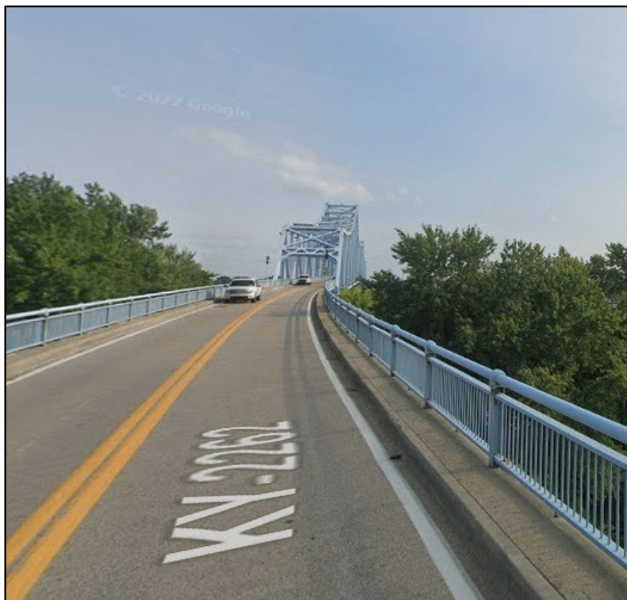
Bridge approaches looking south
