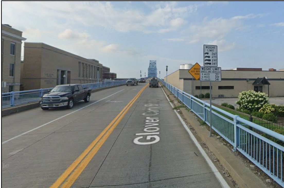
Bridge approaches looking north
