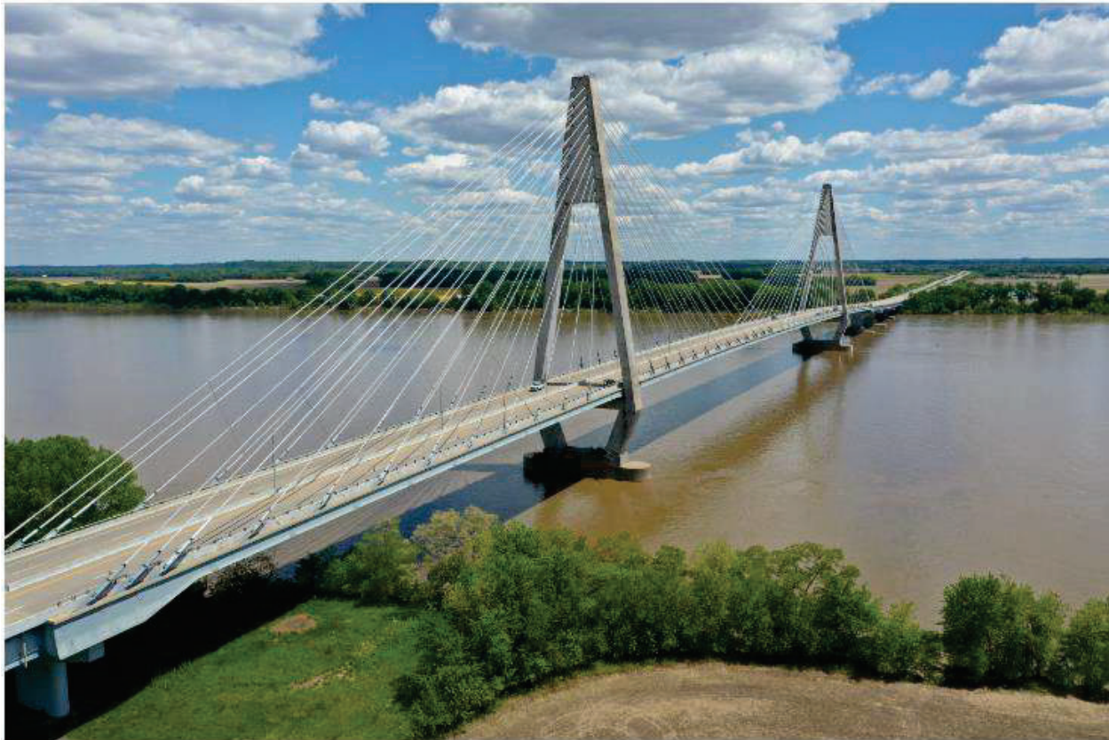
US 231 Bridge over the Ohio River looking towards Kentucky, built in 2002 (KYTC Bridge Inspection database).
