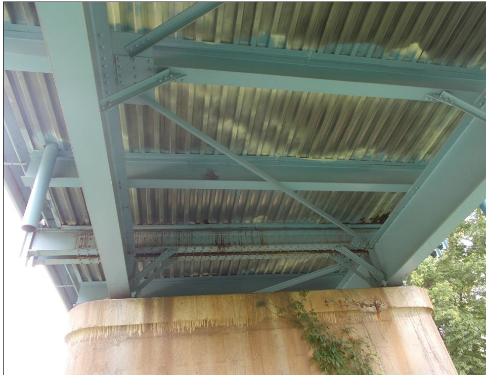
Photo 5: Example of the steel decking under parts of the bridge; August 8, 2023
