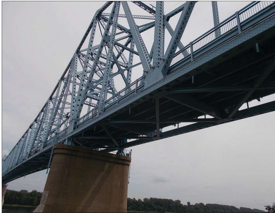
Photo 1: Glover Cary Bridge over the Ohio River; August 8, 2023
