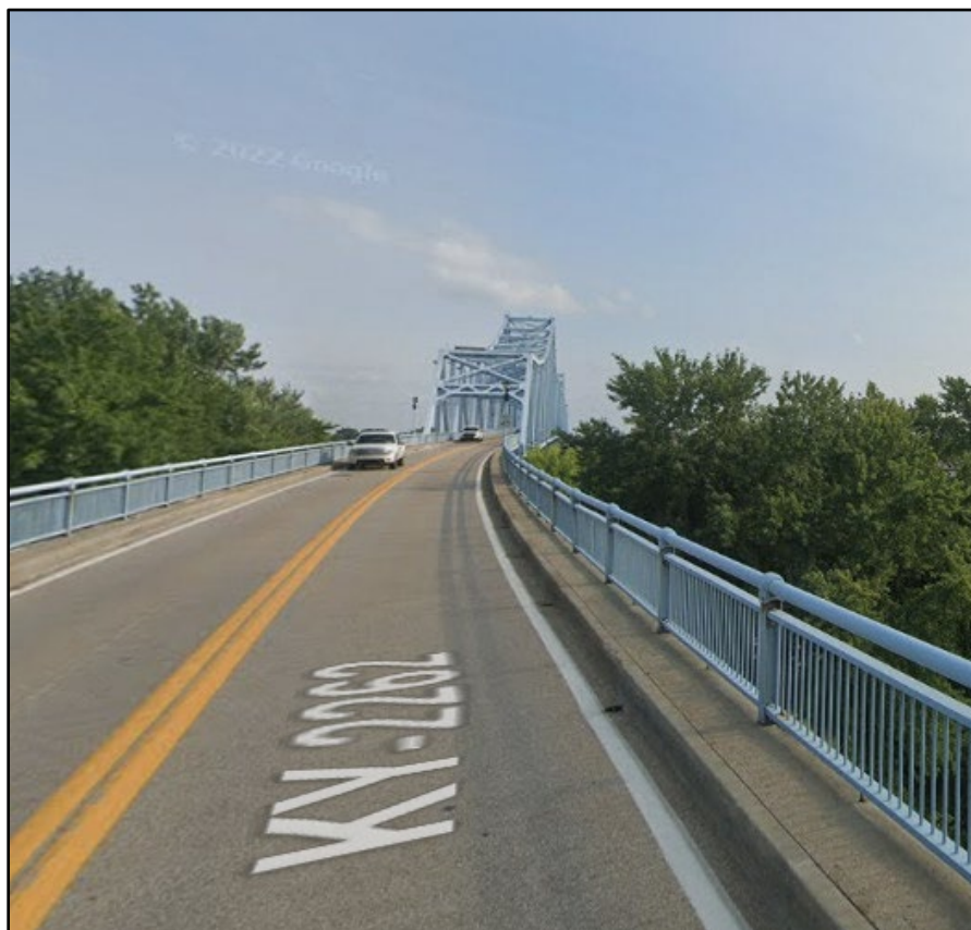
Bridge approaches looking south
