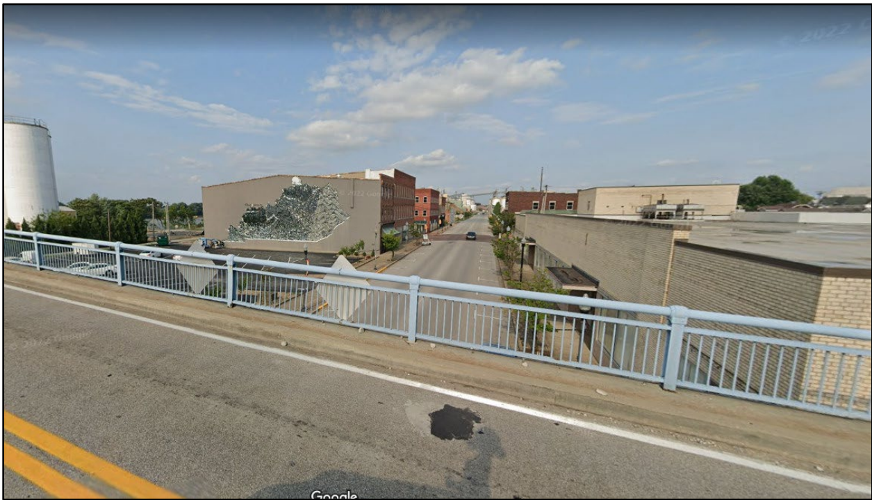
Looking northeast from bridge approaches
