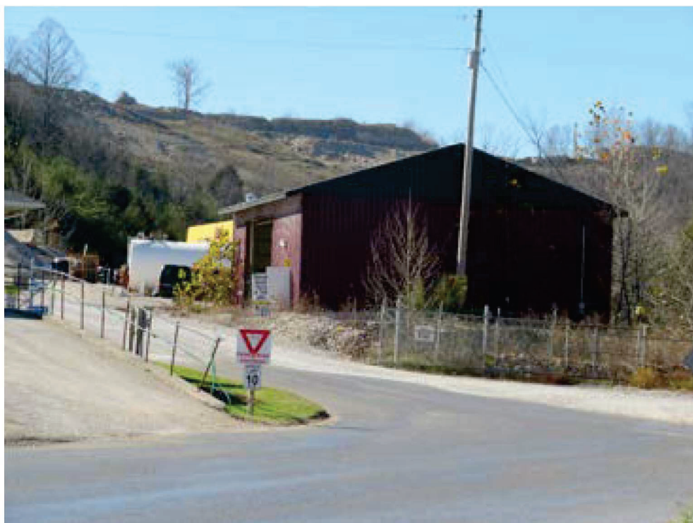
Metal building, looking west.
