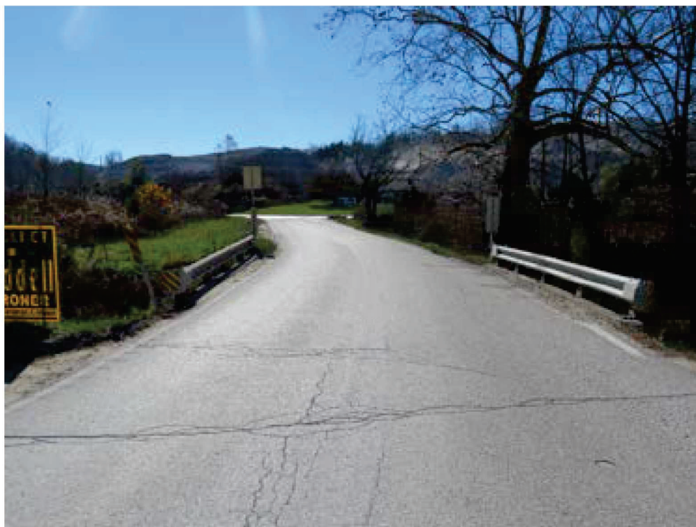
Bridge deck and railings, looking southwest.
