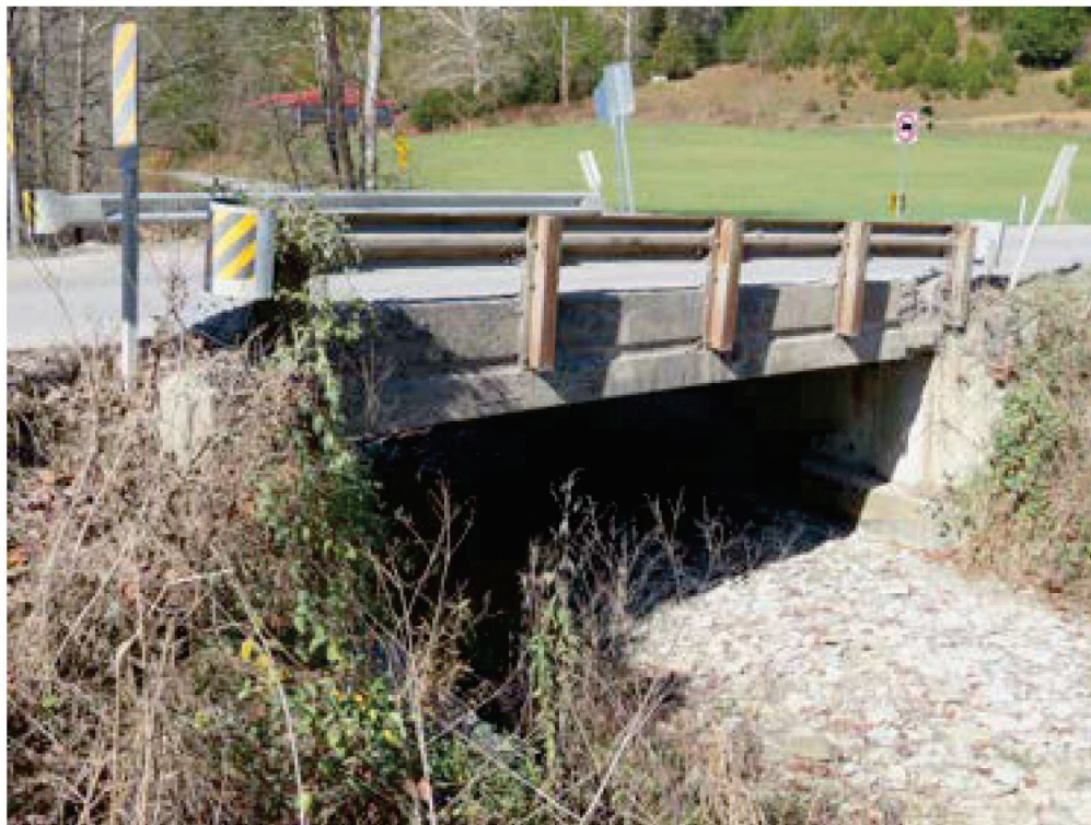
Side view of bridge, looking northwest.
