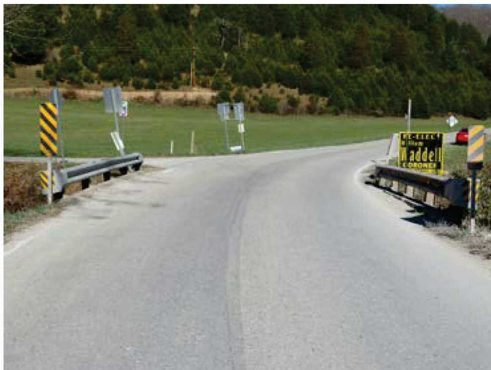
Bridge deck and railings, looking northeast.
