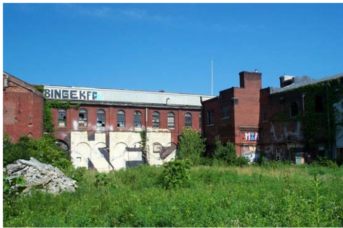
Photograph No. 2 - Left to right view of Buildings 3, 2, and 5 from the courtyard.
