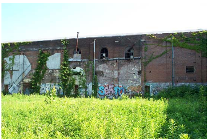
Photograph No. 3 - View of Building 6 from the courtyard.
