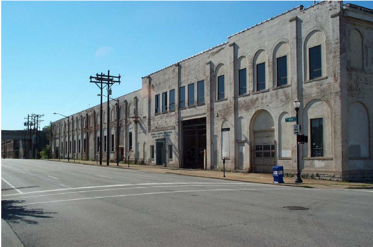
Photograph No. 1 – Left to right view of front of Buildings 6, 5, and 2 from the intersection of Main Street and Jackson Street. The existing highway bridge is shown in the background to the left.
