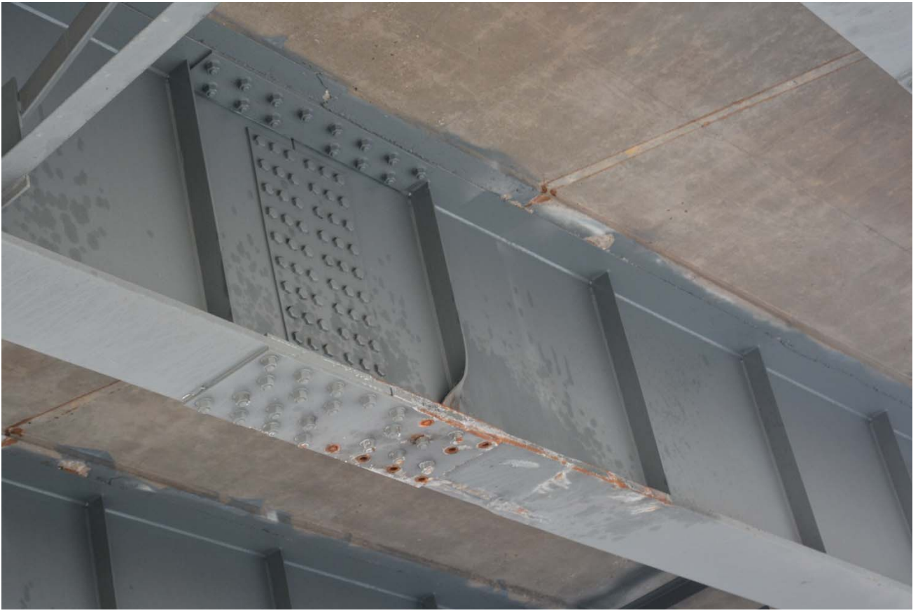
Photo 4- Girder 2 splice – bolt replacement
