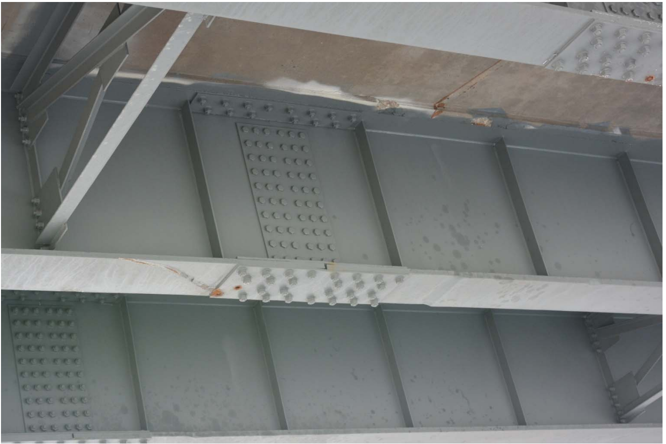
Photo 5 – Girder 3 splice bolt replacement
