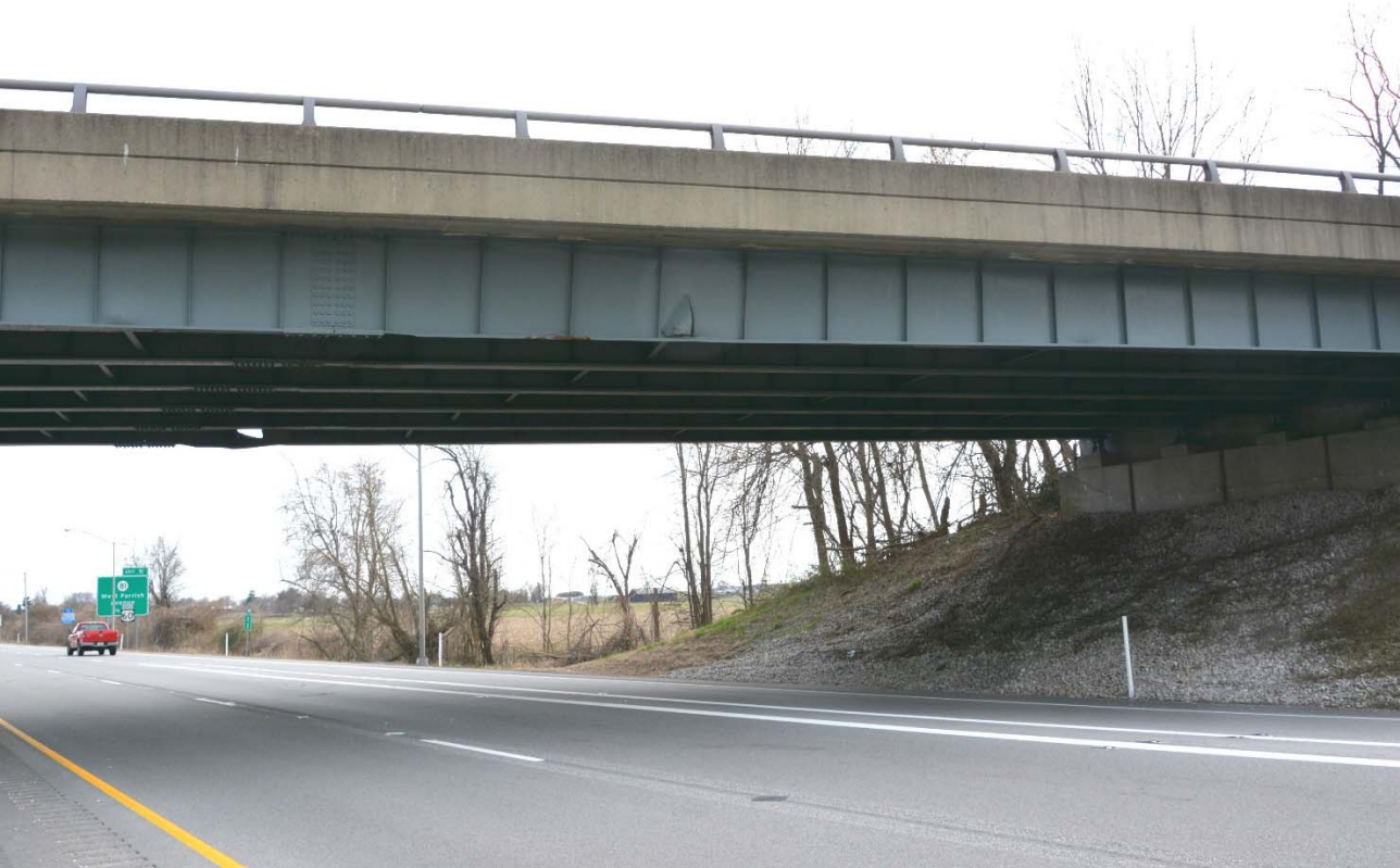
Photo 1 - Girder 1 Heat Straightening area looking toward south from median
