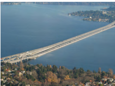
The I-90 floating bridge.
