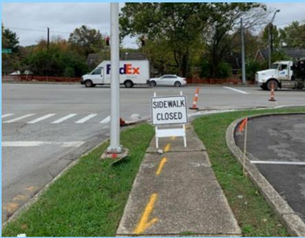
**Figure 9.9** Work zone accommodations for pedestrians on Versailles Road in Lexington, KY.
