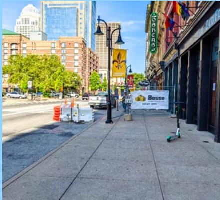
**Figure 9.10** Incorrect and unsafe MOT procedure for pedestrian access, with sidewalk blocked by signage and no clearly identified accessible alternate route around the work zone on US 31W (W. Main Street) in Louisville, KY.
