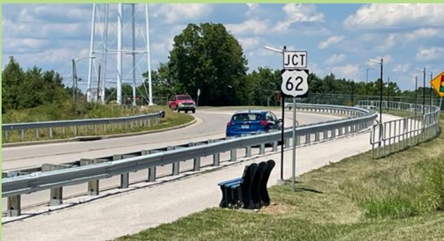
**Figure 9.5** Shared-use path along KY 1448 (Mapleleaf Road) in Maysville, KY with a barrier separation between the path and the motor vehicles and a safety railing protecting path users from steep slopes.
