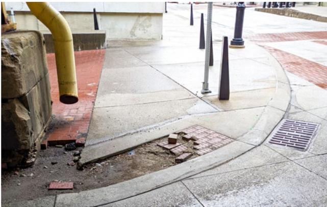
**Figure 6.3** Inaccessible detectable warning pavers on 2nd Street in Louisville, KY.
