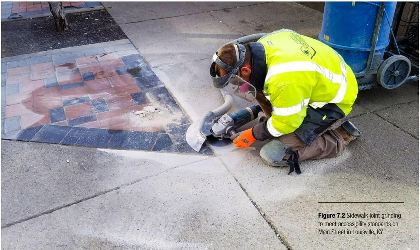
**Figure 7.2** Sidewalk joint grinding to meet accessibility standards on Main Street in Louisville, KY.
