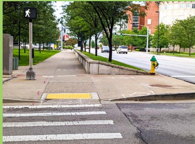
**Figure 5.6** Barrier preventing pedestrian crossings in undesignated locations on S. Limestone in Lexington, KY.
