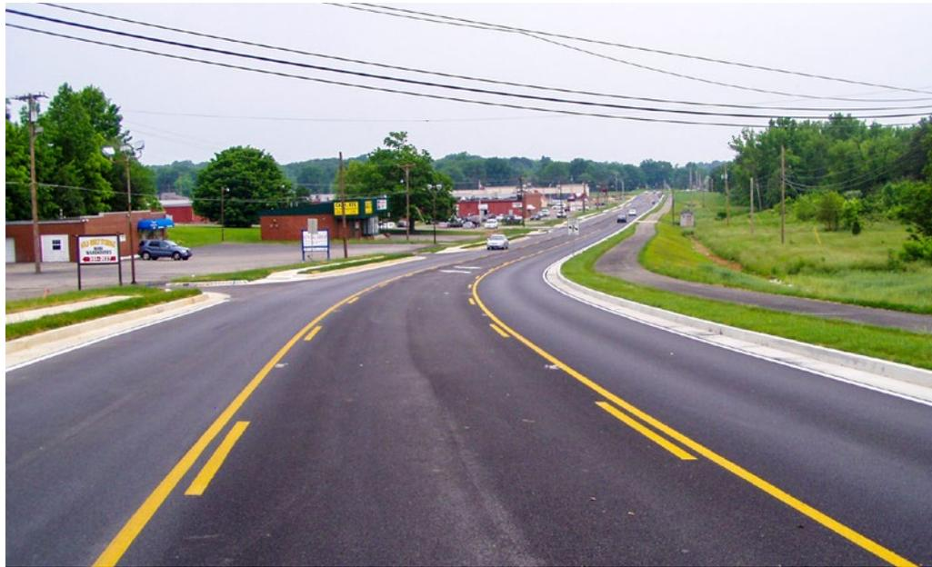
**Figure 7.1** Conversion of Wilson Road in Radcliff, KY from two motor vehicle lanes with no pedestrian or bicycle facilities (top) to include center two-way left-turn lane, sidewalk on the left, and shared-use path on the right (bottom).
