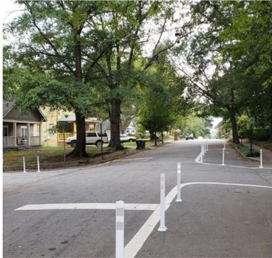
A curb extension is a traffic calming measure that widens pedestrian space on the street by narrowing the roadway. Tactical curb extensions are made of low cost, quick build materials such as striping, vertical delineators, and paint.
