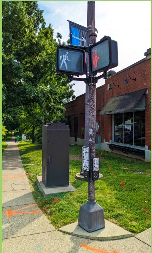
**Figure 6.9** Pedestrian signals and push buttons at the corner of US 60A and US 150 in Louisville, KY.
