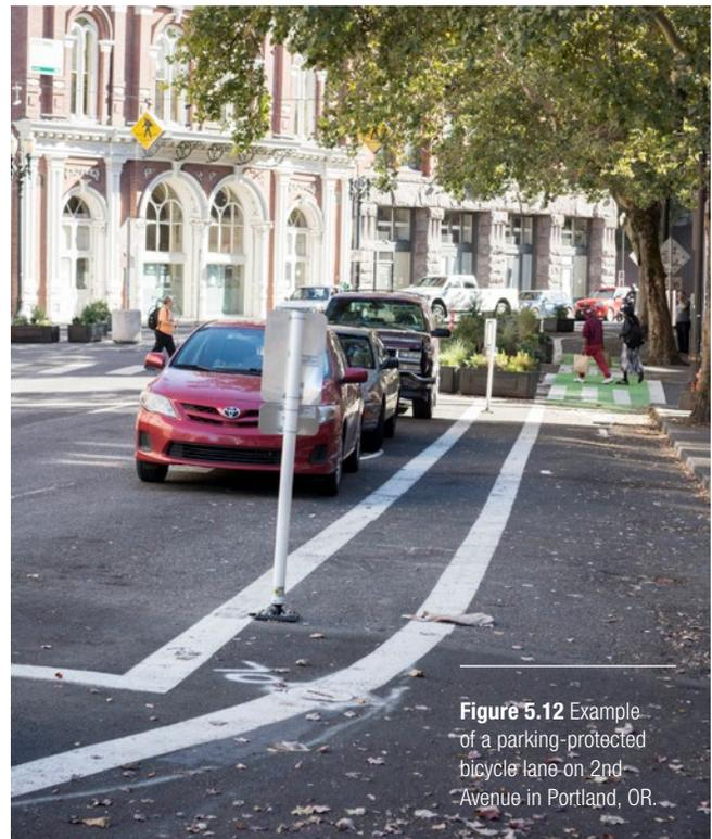
**Figure 5.12** Example of a parking-protected bicycle lane on 2nd Avenue in Portland, OR.
