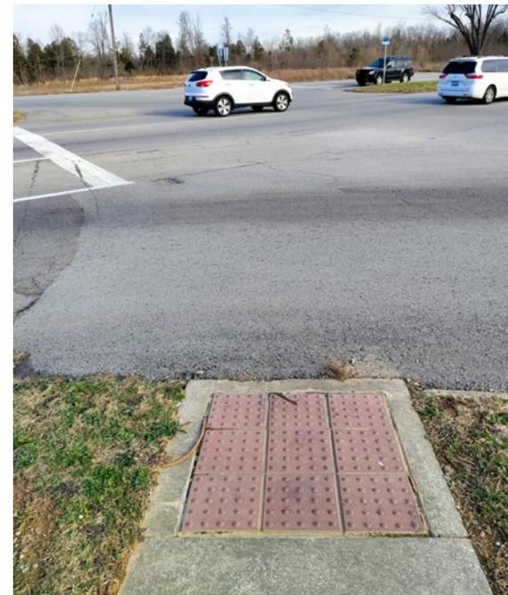
**Figure 4.1** Incorrect ramp and detectable warning alignment, pointing the pedestrian toward the middle of the intersection.
