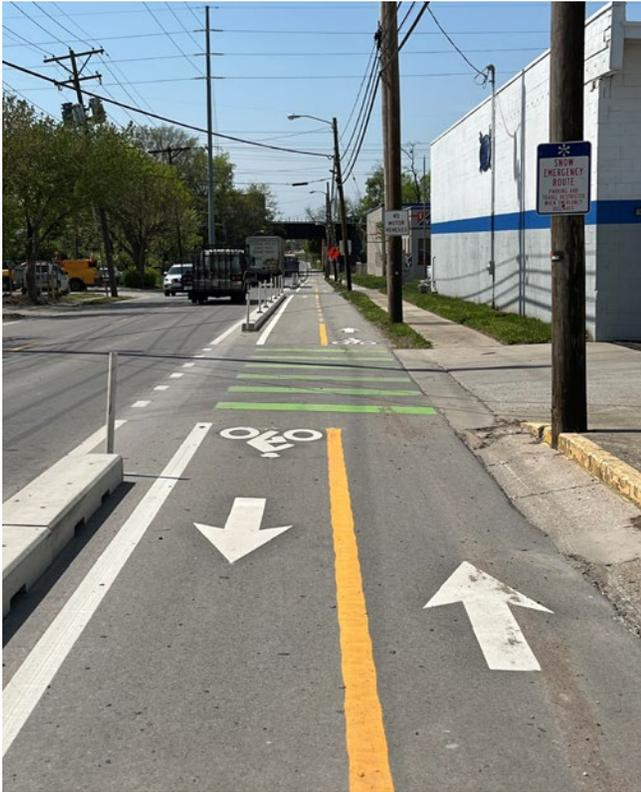
**Figure 5.19** Separated two-way cycle track on Manchester Street, Lexington, KY.
