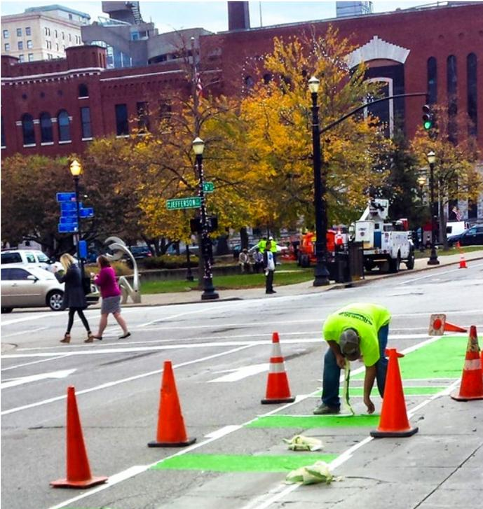
**Figure 9.8** Contractor placing MMA green pavement markings on 6th Street in Louisville, KY.
