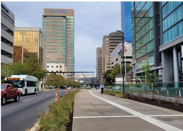
**Figure 5.20** Two-way cycle track (left) and pedestrian path (right) separated by a concrete band on Town Branch Commons in Lexington, KY.
