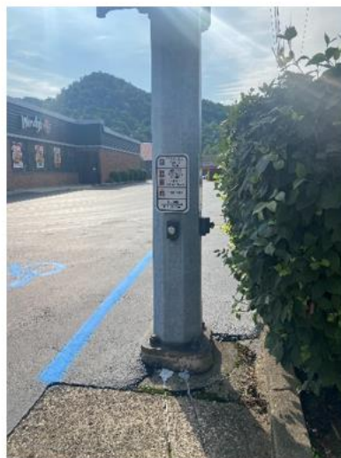
Figure 38. Inaccessible pedestrian push buttons.
