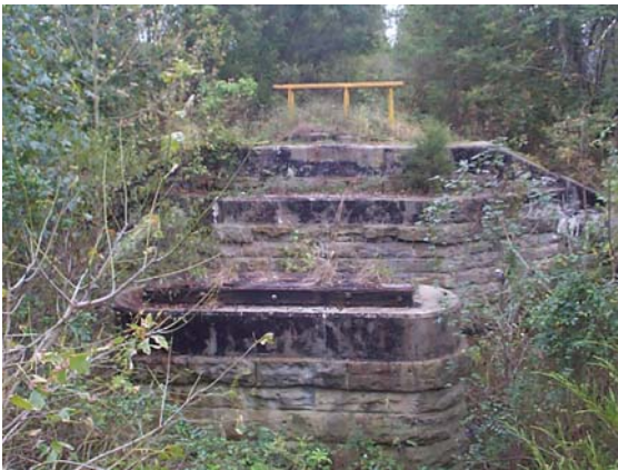
Bridge supports on former Lebanon Branch near Crab Orchard
