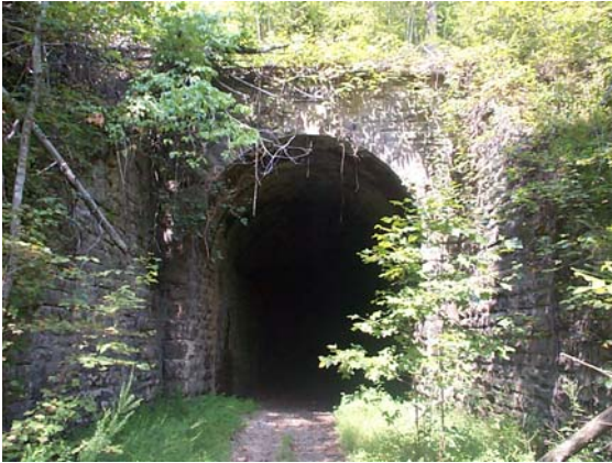
Tunnel south of Burnside on former CNO&TP
