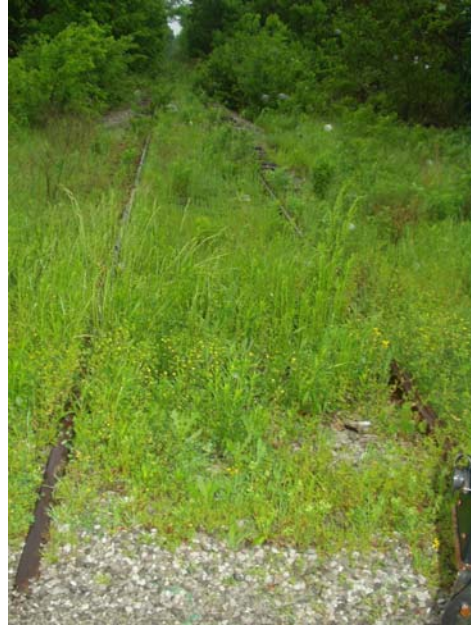
Rails on the ground near Princeton
