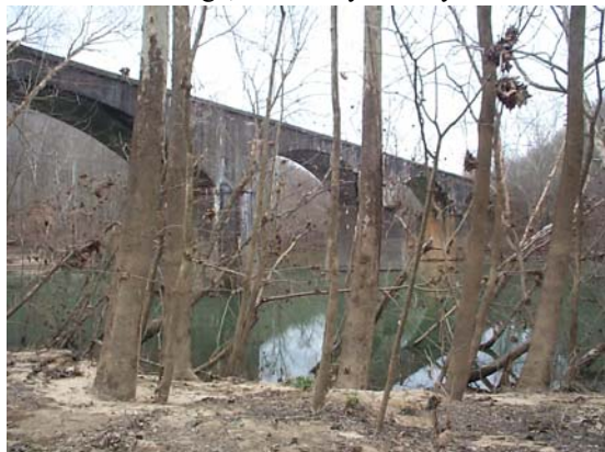
Yamacraw Bridge, McCreary County
