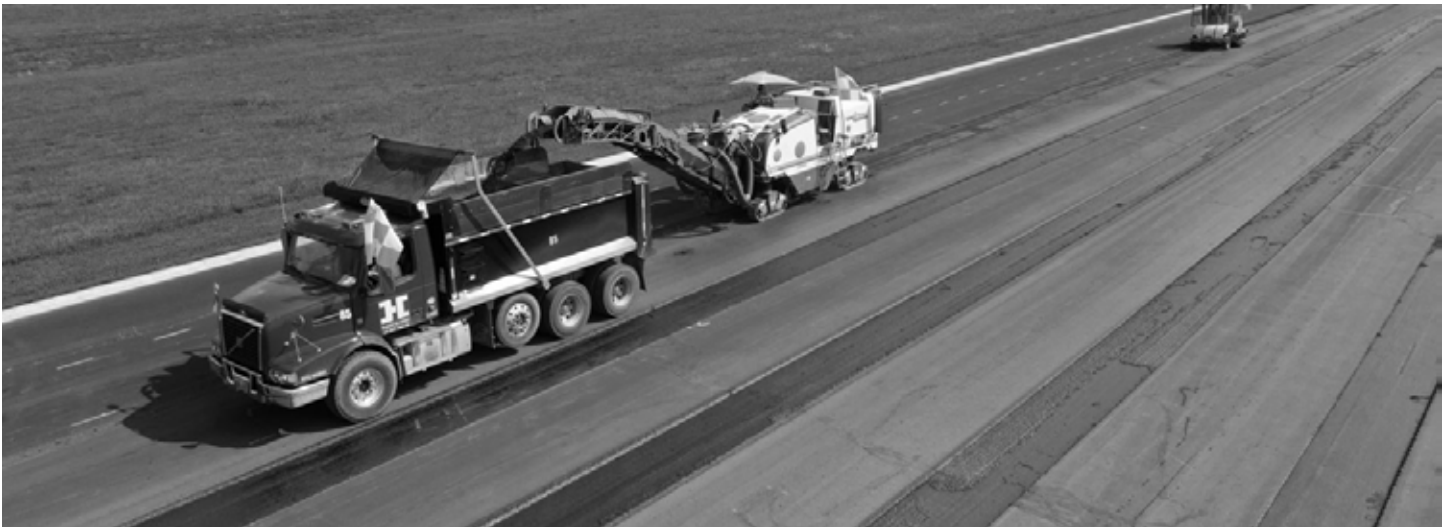
Contractors work on runway at Kentucky airport.
