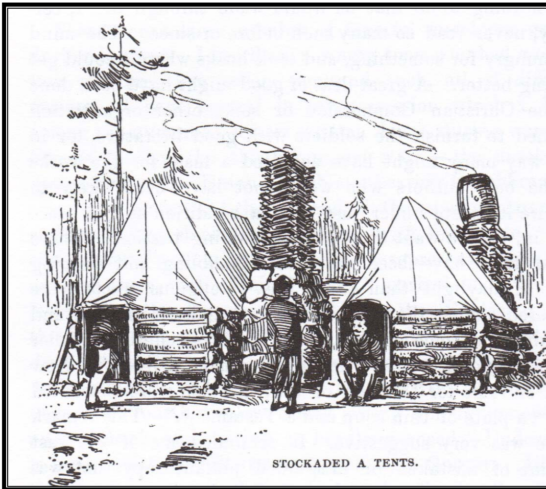
Figure 12. Illustration of a Stockaded Tent or Winterized Shelter (Billings 1993).
