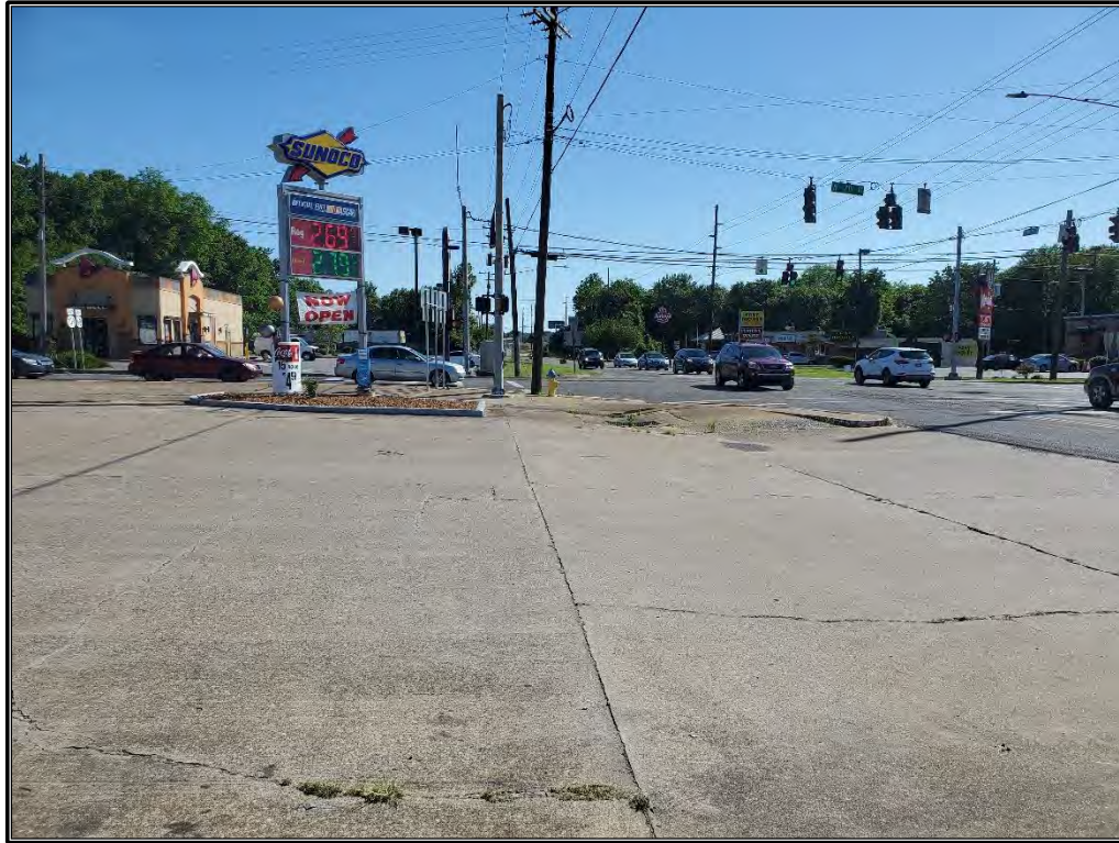
Figure 9. Overview of the project area within a paved lot, facing southwest.
