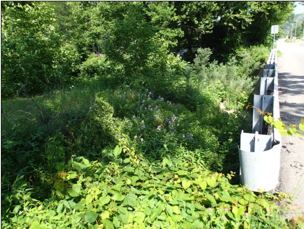
Figure 3-6. View of APE south side of KY 474, sloped and disturbed with ditch, road, and creek improvements, looking east southeast.
