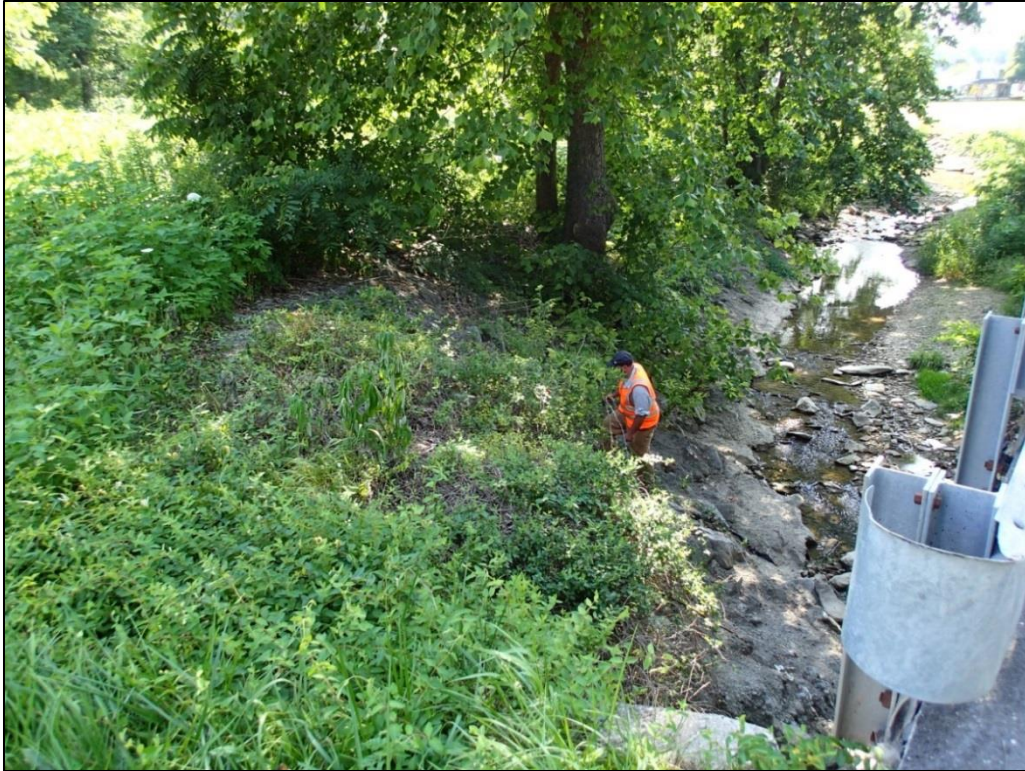
Figure 3-7. View of APE, south side of KY 474, along Smith Creek. Sloped and disturbed by erosion and shoring-up/graveling for road/bridge reinforcements.
