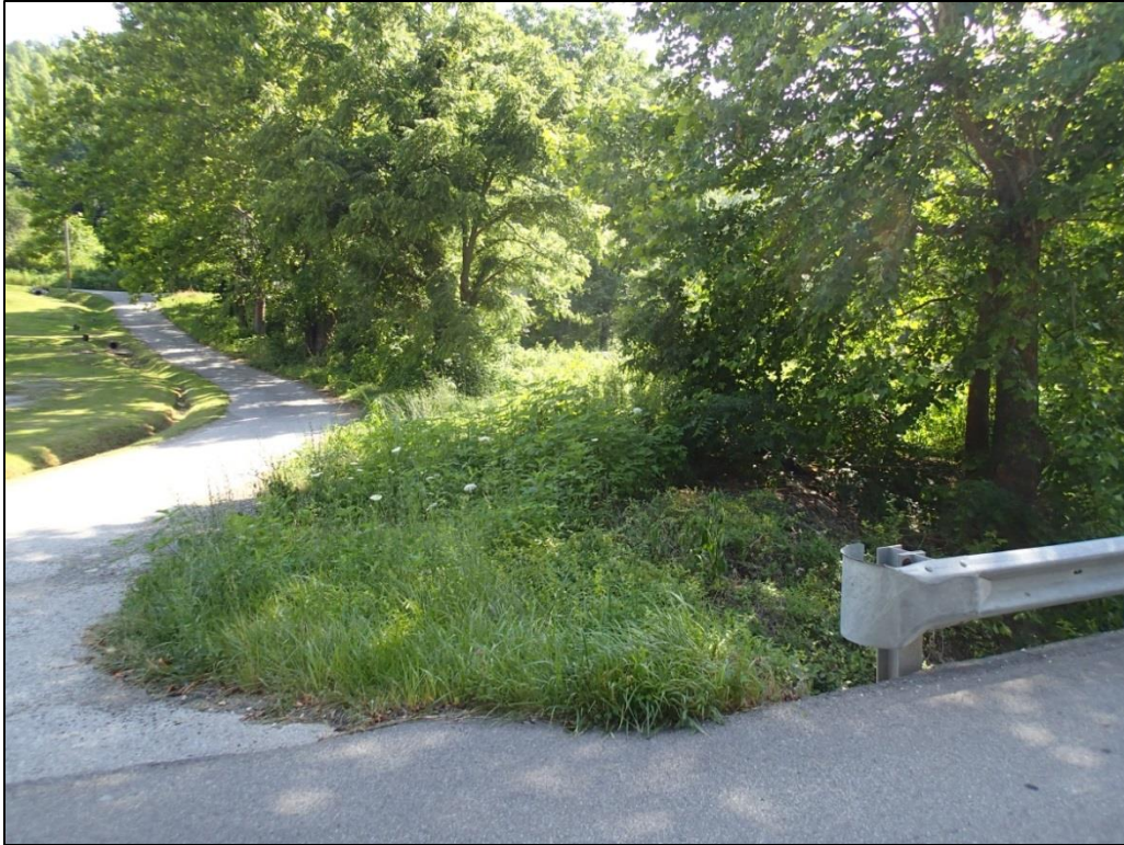
Figure 3-9. APE along Nunn Road, disturbed with road and ditch construction, looking south southwest.
