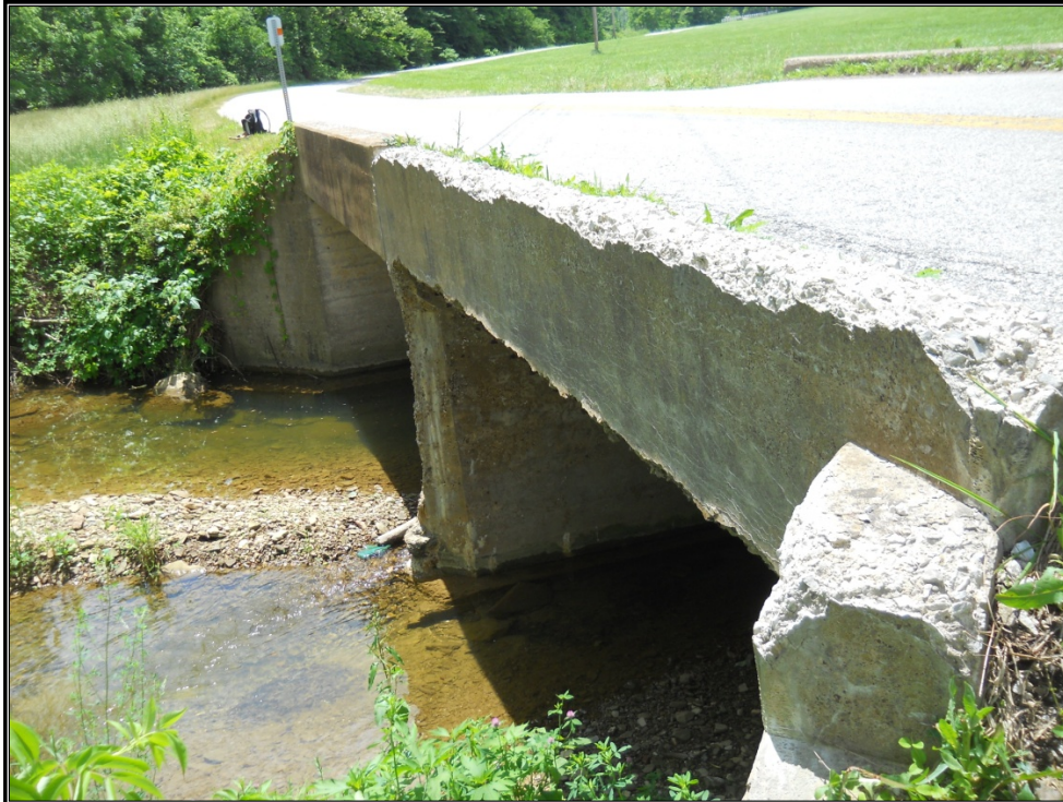
Figure 7. Detailed view of existing bridge, facing south.
