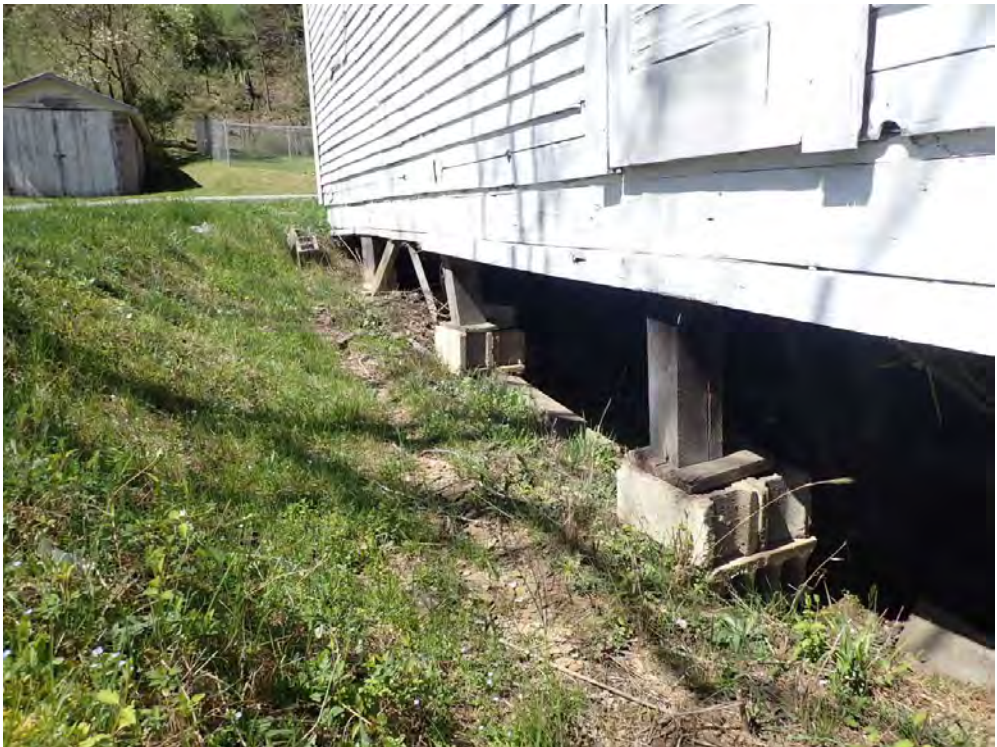
Figure 34. Piers under building.
