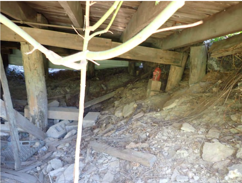
Figure 36. Fill at rear of building.
