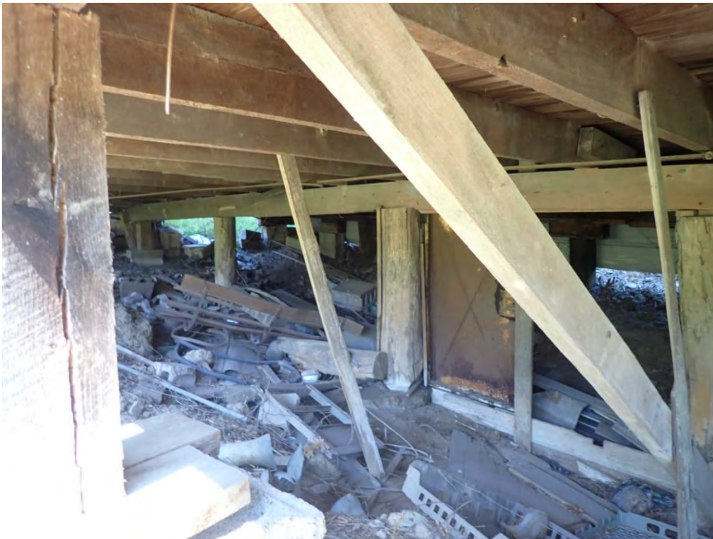
Figure 35. Original grade sloping upward to front of building.
