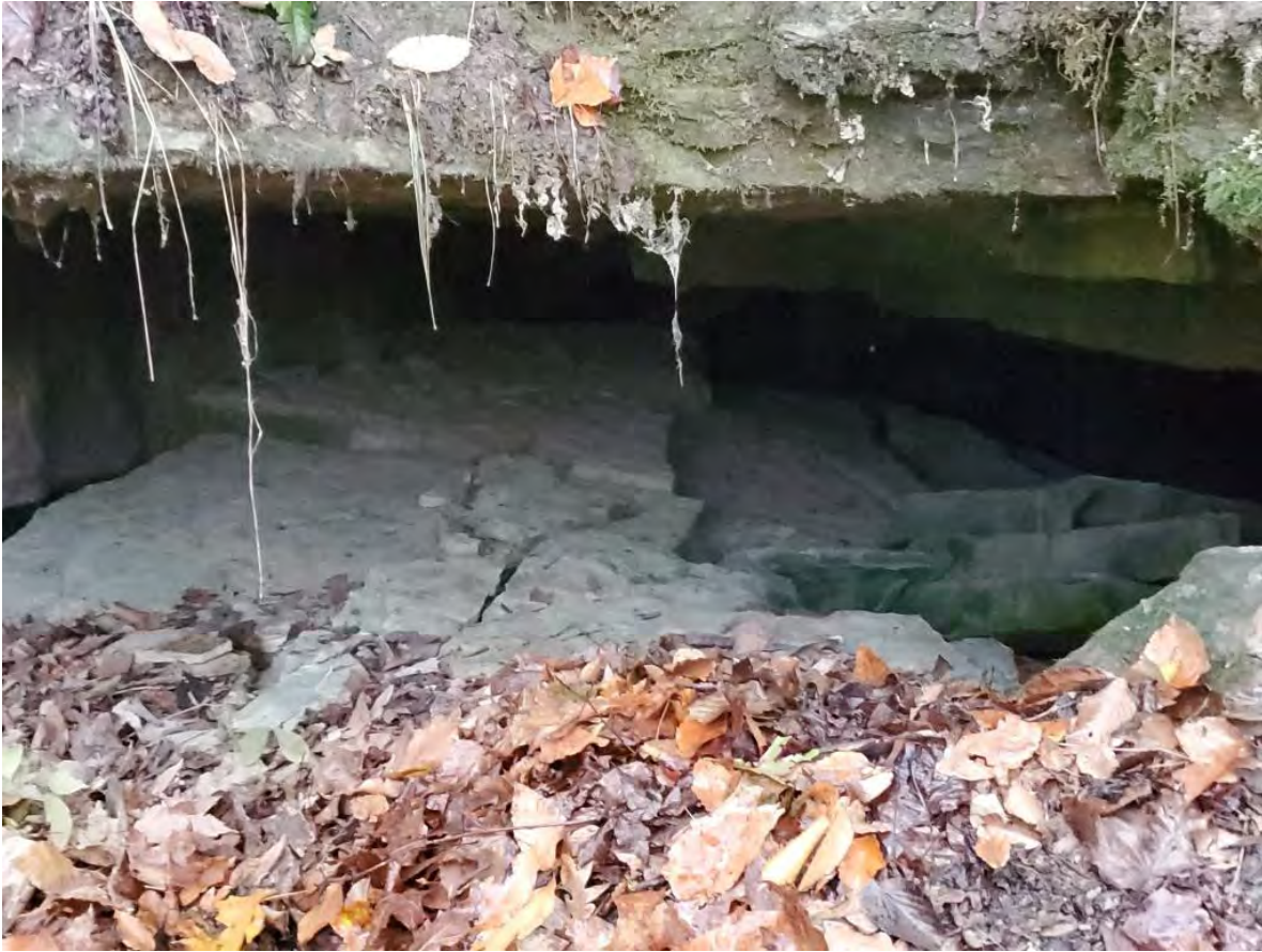
Figure 73. Mine portal interior.
