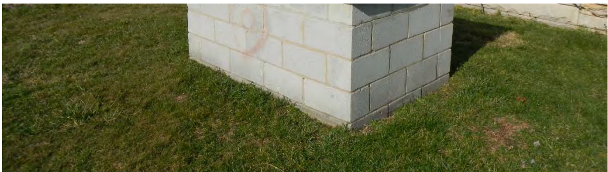
Figure 73. Overview of well house at Site 15Mo174, facing northeast.
