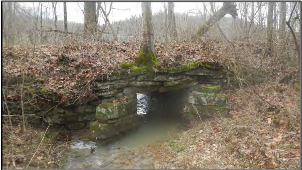
Figure 21. Overview of stone culvert in the project area, facing south.
