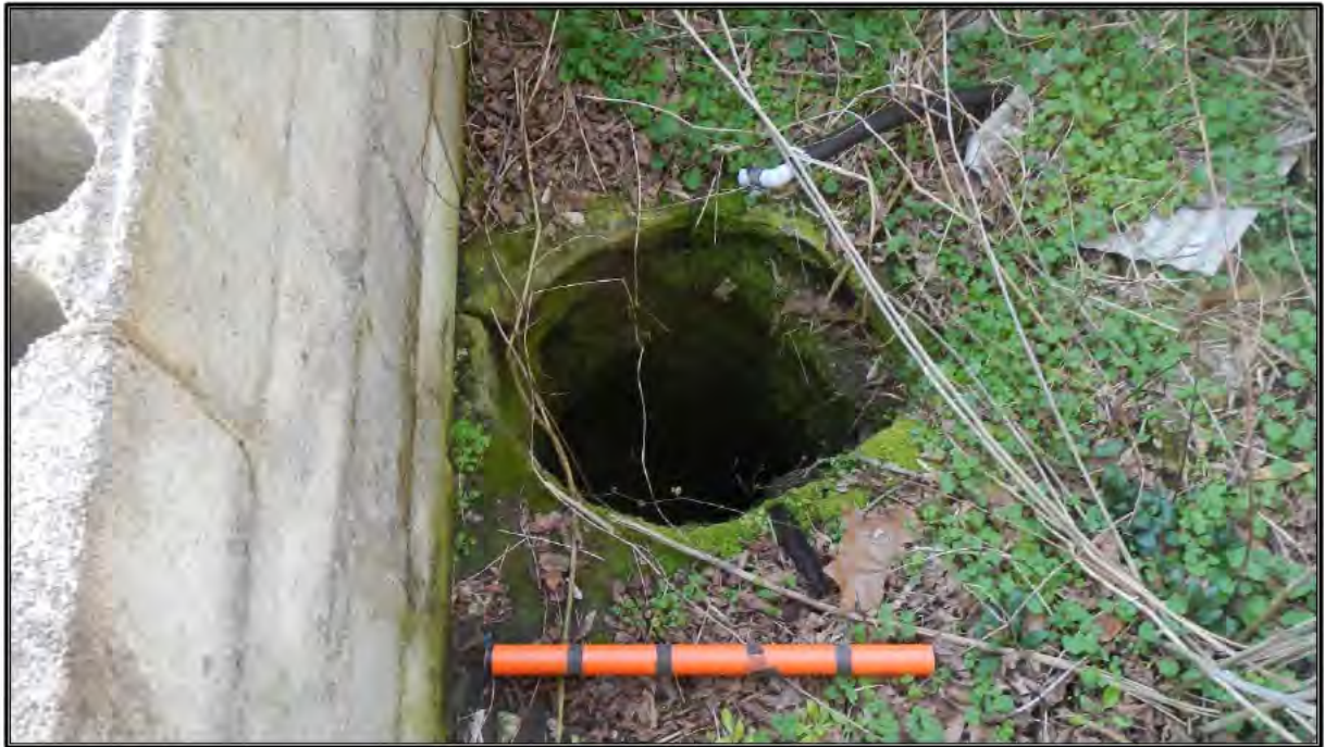
Figure 64. Limestone block well at Site 15EI81.
