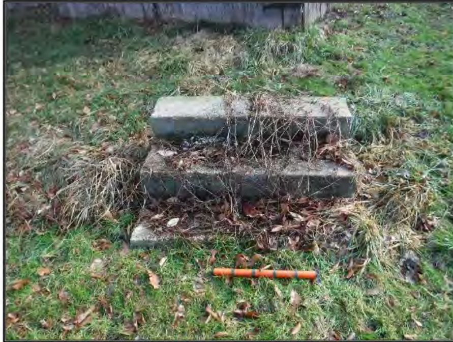
Figure 91. Concrete steps present at Site 15Mo176, facing east-northeast.
