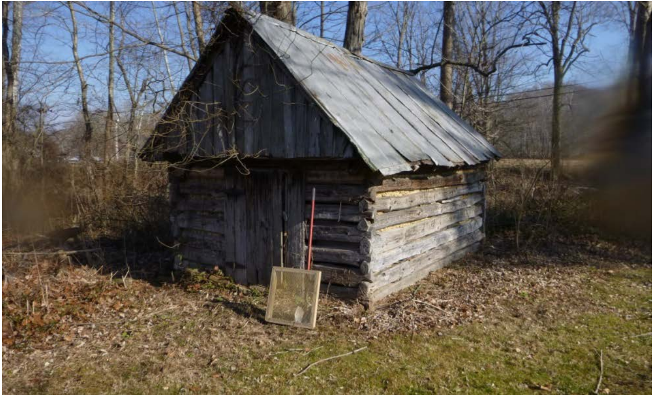
Figure 6.31. Structure 3, a Small Log Outbuilding (looking northeast).
