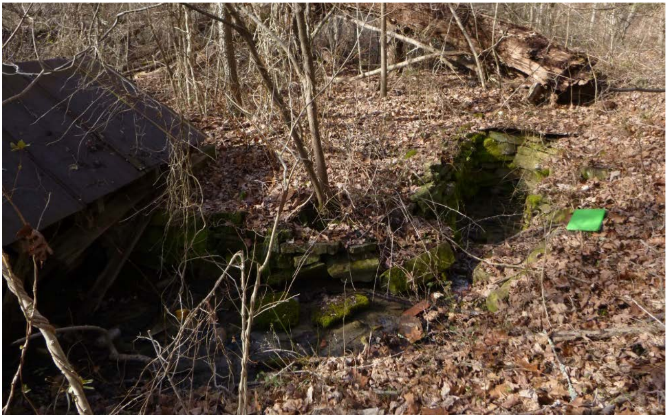
Figure 6.22. Keyhole Stone Springhouse Foundation at 15Ro230 (facing south).
