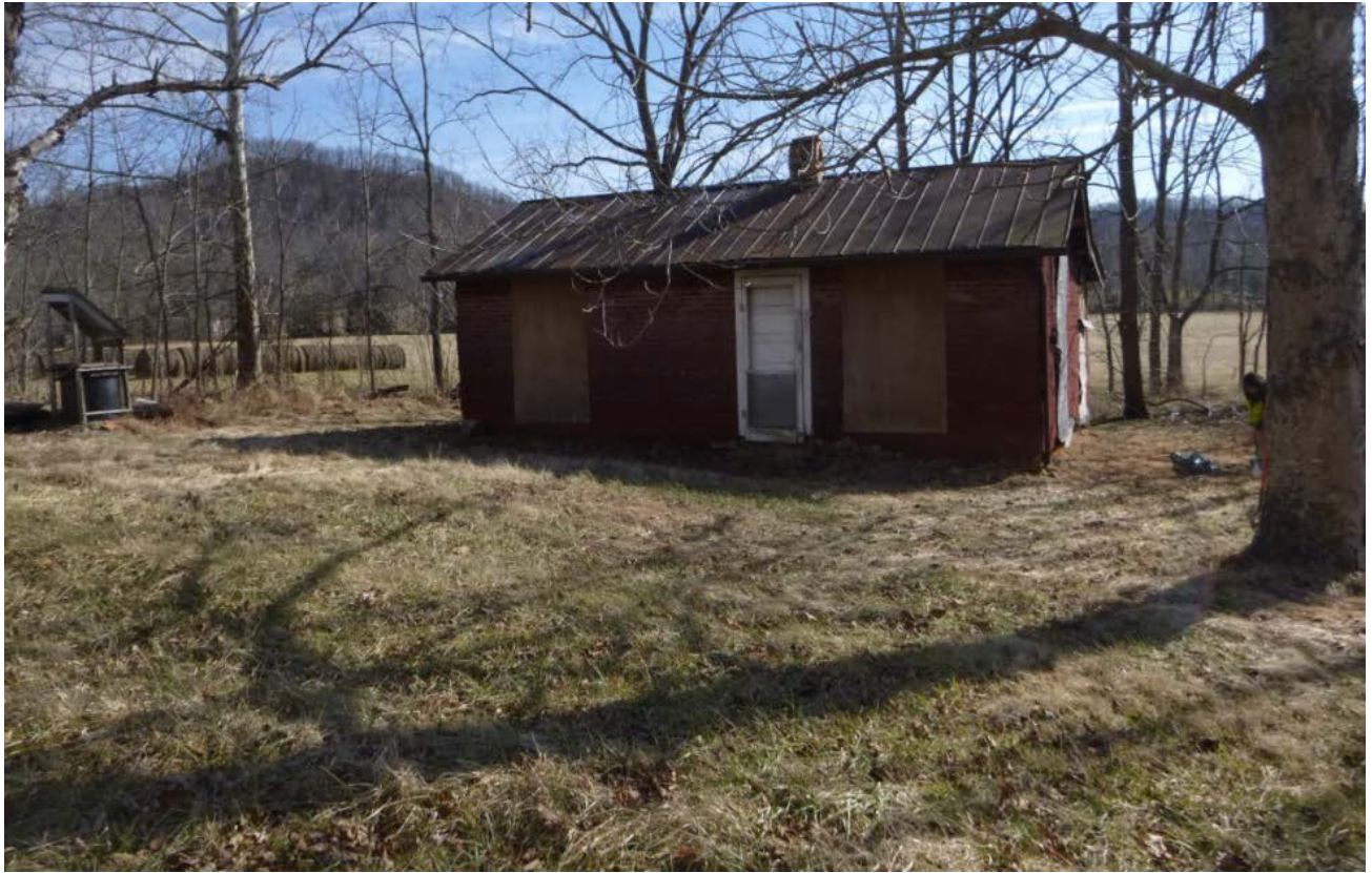
Figure 6.27. Structure 1 House and Well (looking east).
