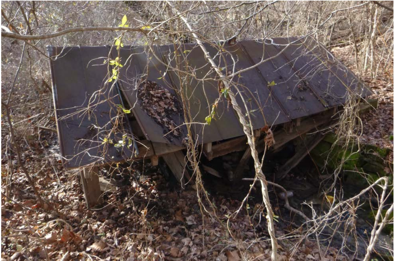
Figure 6.21. Collapsed Wooden Springhouse Superstructure at 15Ro230 (facing southeast).
