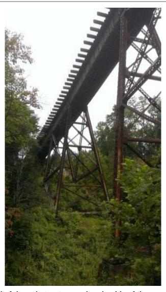
Figure 116. Detail of the substructure and underside of the superstructure of the Howard's Creek Viaduct.
