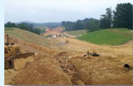
Linear construction sites require special attention to drainage within—and into—the construction zone.
