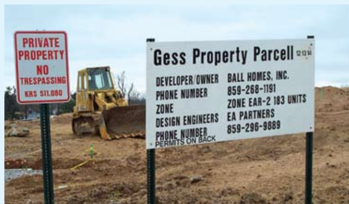
Listing the construction site operator and posting applicable permits makes it easy for inspectors to quickly check whether or not a site is in compliance with various state and federal regulations.
