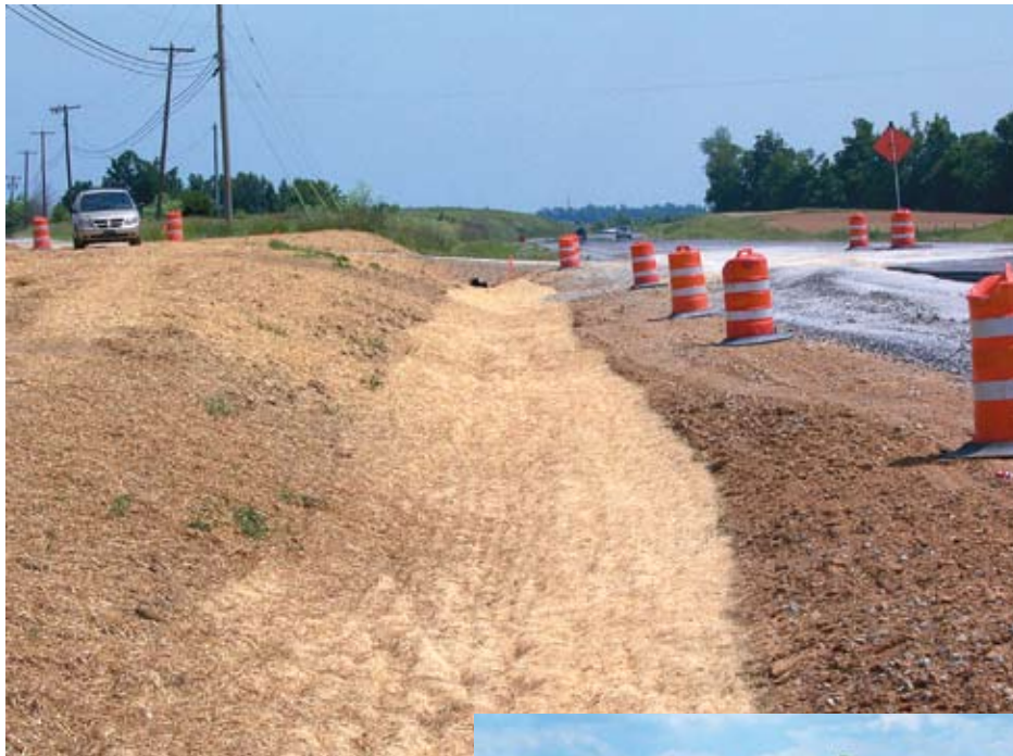
Here is an excellent construction of triple-seeded ditch with excelsior blanket. Ditches should be stabilized, seeded, and mulched immediately after construction.
