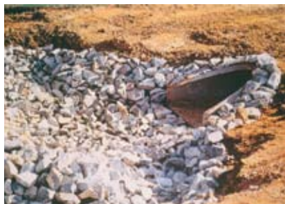
Good example of dissipator apron construction for low tailwater conditions.
