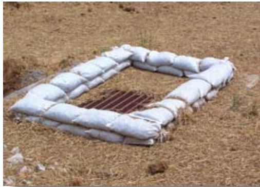
Inlet protection berm constructed of half-filled stone bags. Use #57 rock, overlap bags to eliminate large openings and rapid flow-through.
