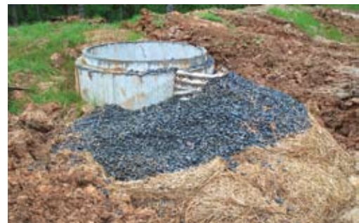
Side hole in drop inlet protected by half-round section of corrugated metal pipe with one-inch holes, held in place by stone berm. This modification can also be used on sediment basin outlet risers.
