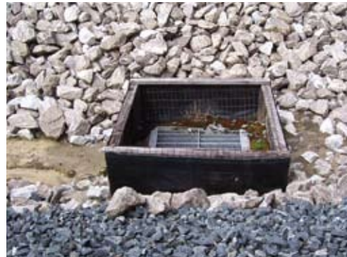
Silt fencing can be used as an inlet protection device if flow volumes and velocities are low. When using a silt fence frame to construction in inlet protection dike, add wire reinforcement and cross-bracing to prevent collapse in areas of heavy flows.
