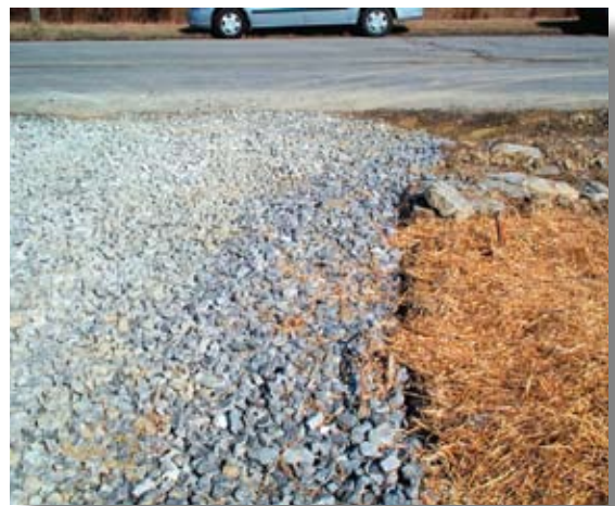
The construction exit will be one of the first things an inspector sees at the construction site and is often a good indication of how other controls are installed and maintained.
