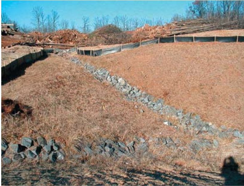
Install silt fencing, sediment traps, and stabilize ditches before clearing and grading. Make sure stakes are on the downhill side of the silt fence!
