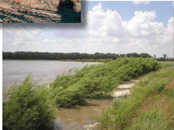
Flag off and preserve vegetated areas along streams, wetlands, lakes, and ponds wherever possible. Keeping these areas intact minimizes the expenses involved in CWA section 404 permitting and extensive erosion and sediment controls. Watershed vegetation provides an excellent buffer against sediment carried by sheet runoff.
