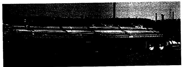
3. Cover the bars or bundles with opaque polyethylene sheeting or other suitable protective material. For stacked bundles, drape the protective covering over the sides of the bundles around the perimeter of the stack. Secure the covering adequately, and make provisions for adequate air circulation around the bars to prevent condensation under the polyethylene sheeting.
