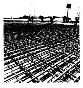
tron Workers Completing Placement of Coated Bars In Large Bridge Deck
