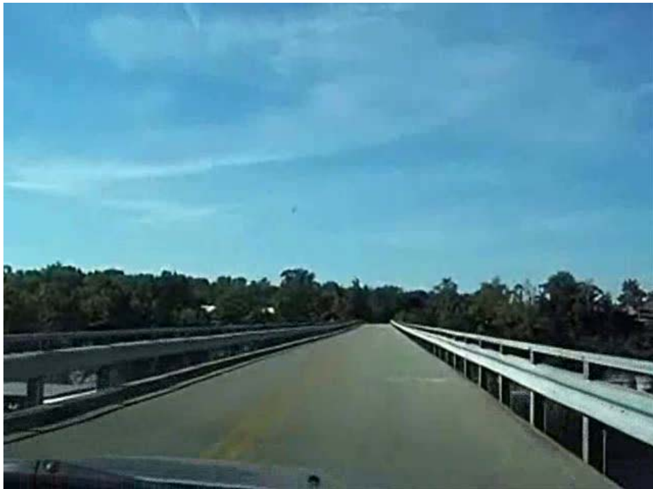
Figure 3: Roadway on Herrington Lake Bridge
