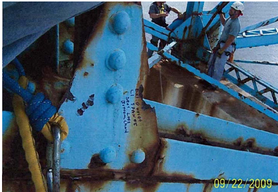
Figure 5: Structural condition of the bridge in 2009
