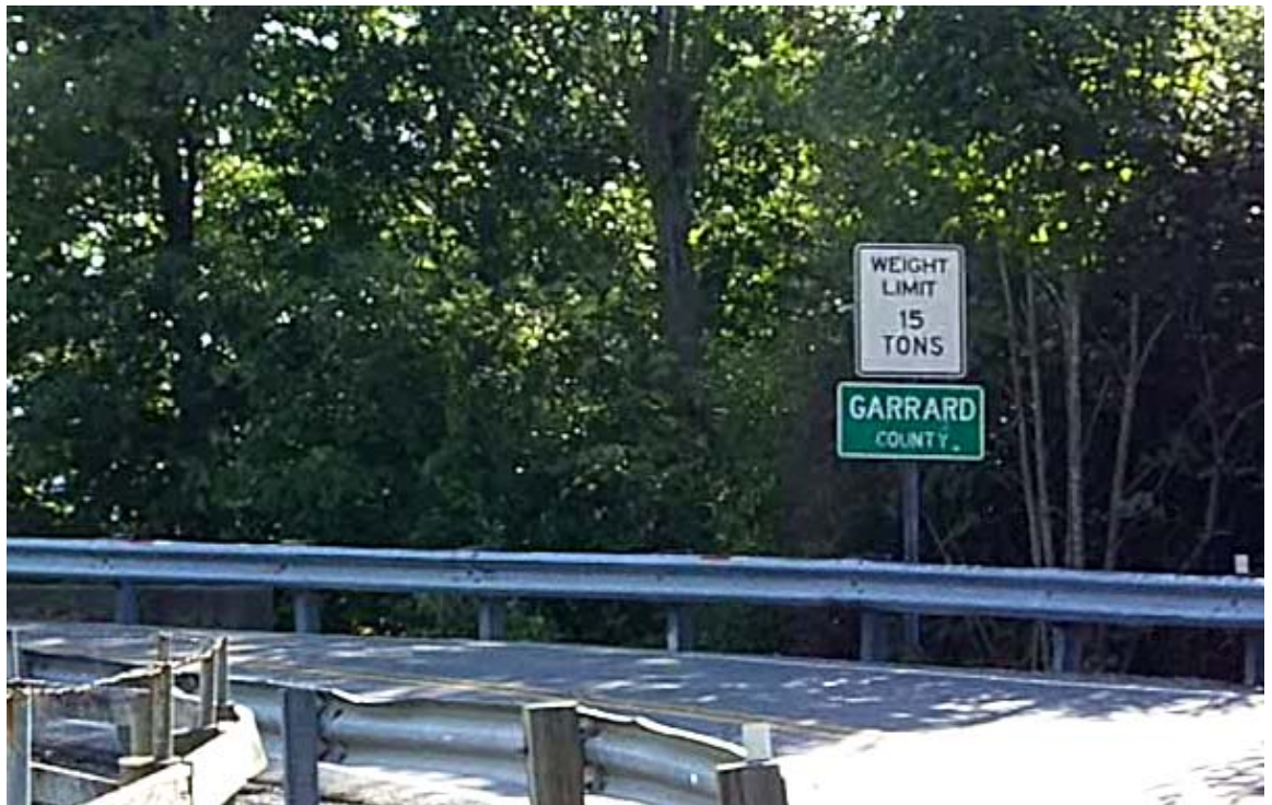
Figure 7: Current posted weight limit on the bridge is 15T
