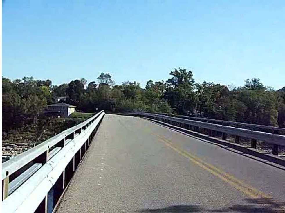
Figure 4: Roadway on Herrington Lake Bridge at the West End
