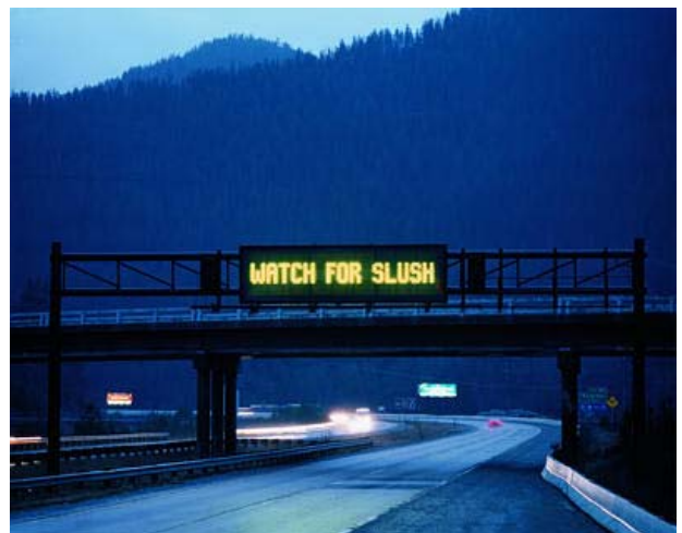
Message Signs Improve Driver Awareness
