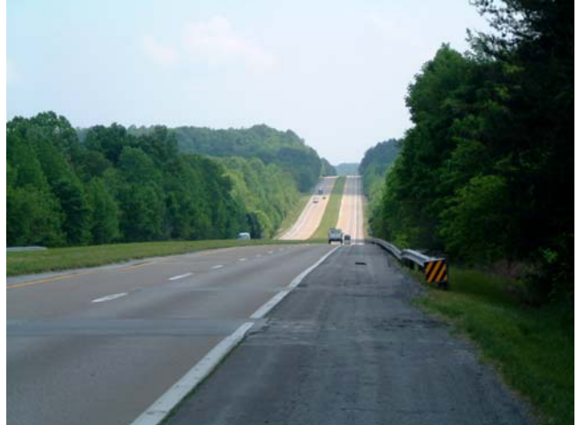
Milepoint 32.733 in Hopkins County along the Ford Parkway was one of five locations identified where the vertical curve is less than the calculated minimum.
