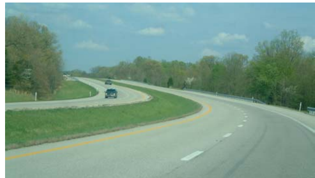
Median widths along the parkways range from 30 to 45 feet.
