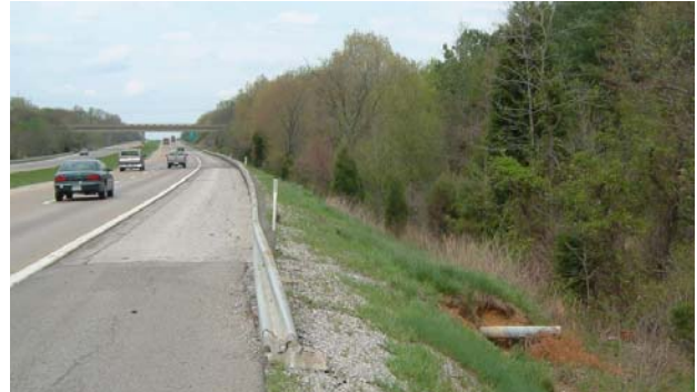
Clear zones and guardrail placement may require upgrades at many locations along the parkways.
