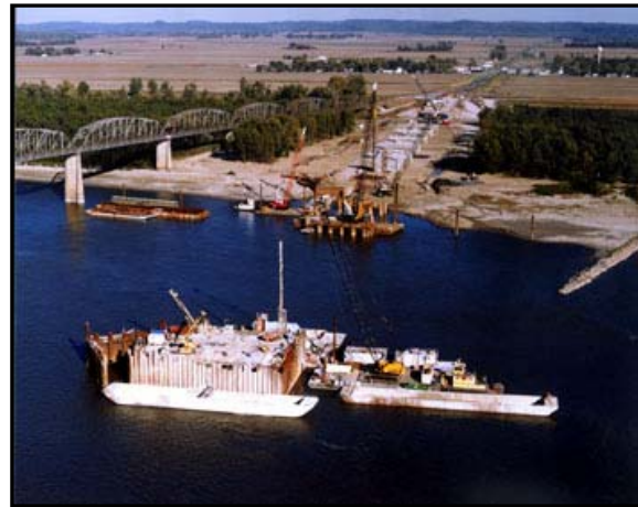
Figure 4. View of Illinois Approach, Cape Girardeau, IL
