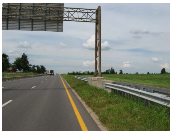
Mayfield Bypass median and inside paved shoulder width does not meet current interstate standard
