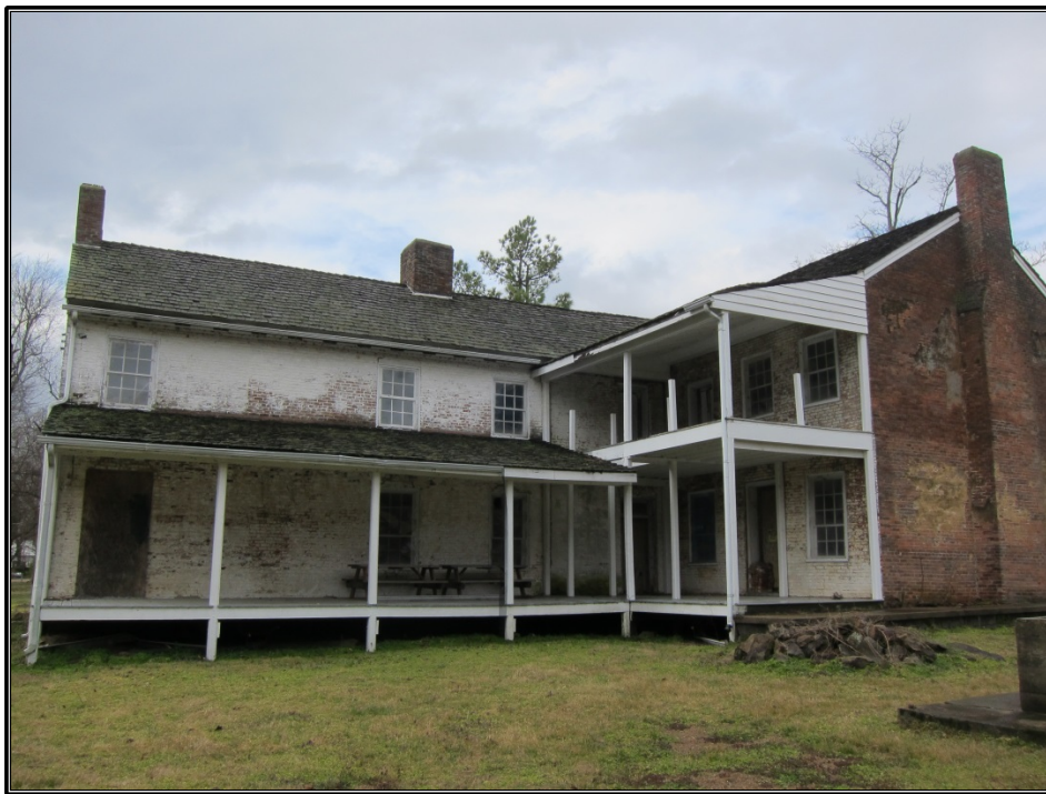
Figure 28. Site 4 (LVS 1): Southwesterly view of the Gower House.
