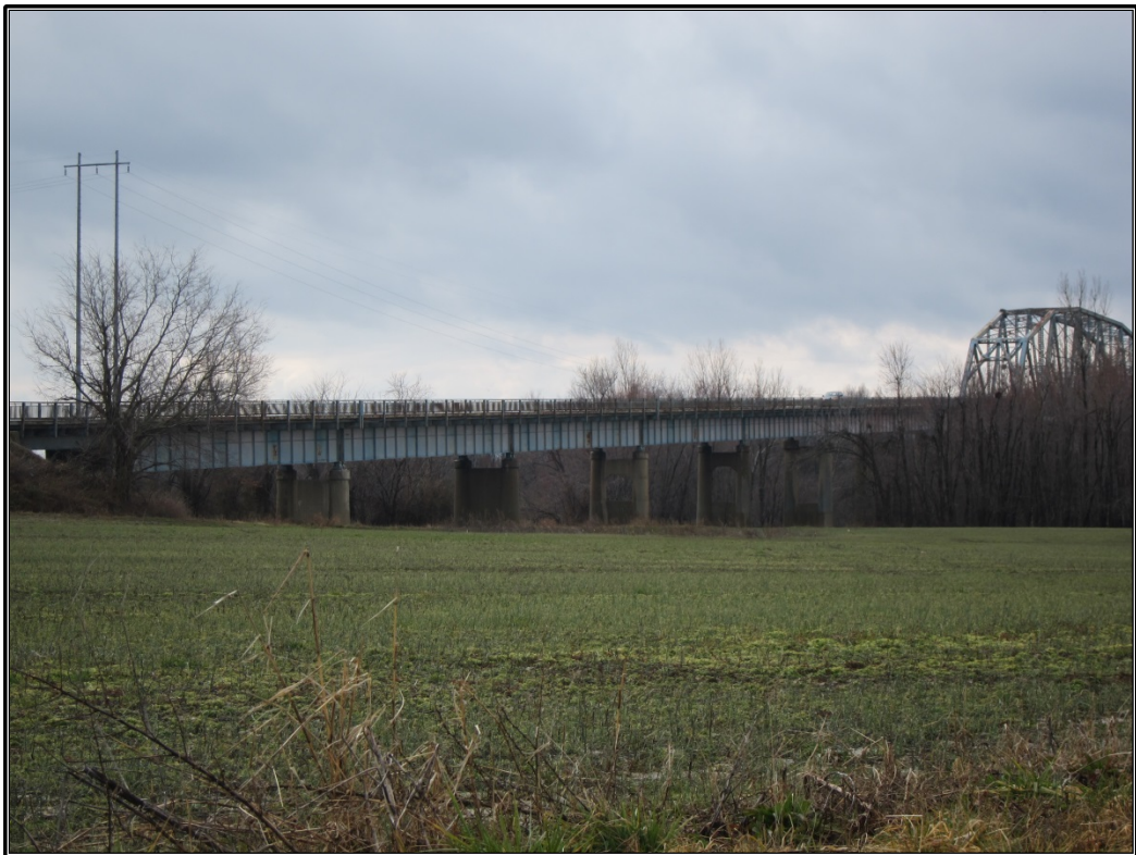
Figure 20. Site 1 (LVS 35): Northern approach span.
