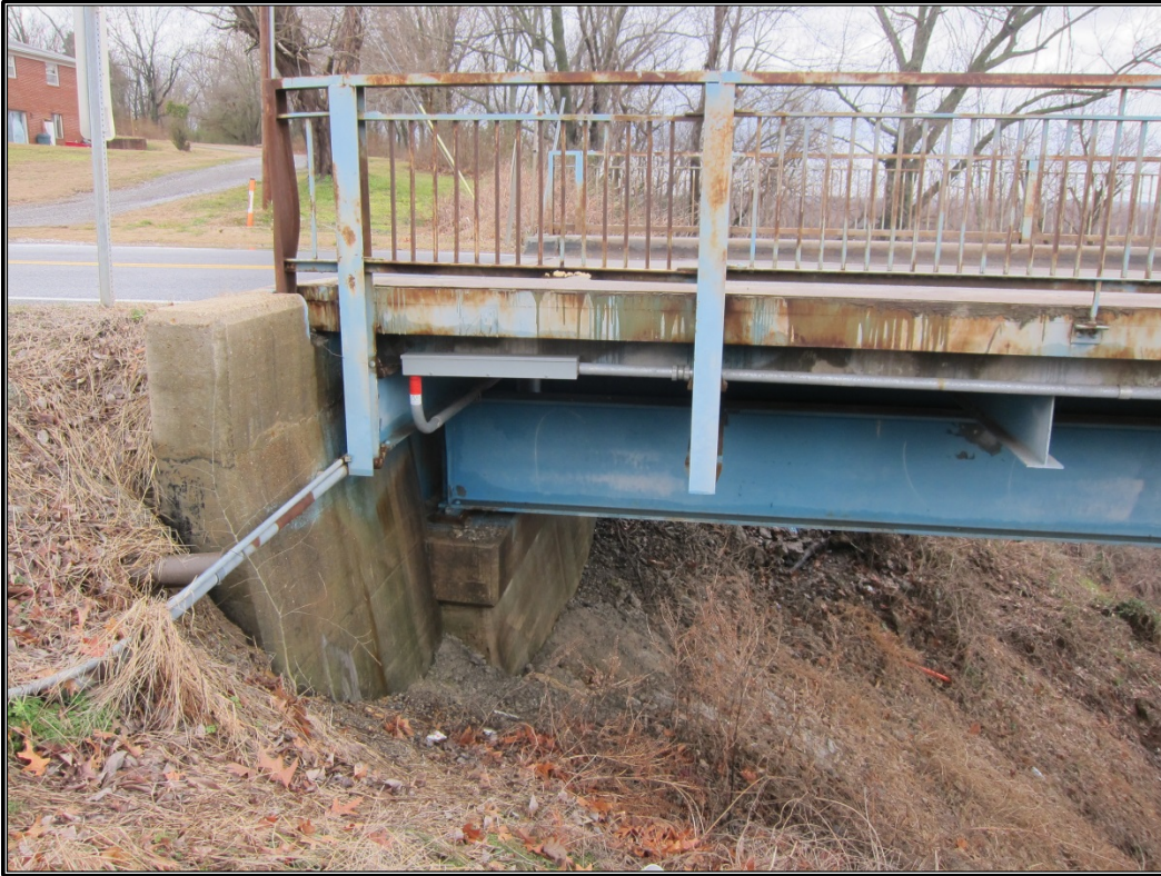
Figure 19. Site 1 (LVS 35): Southern abutment.
