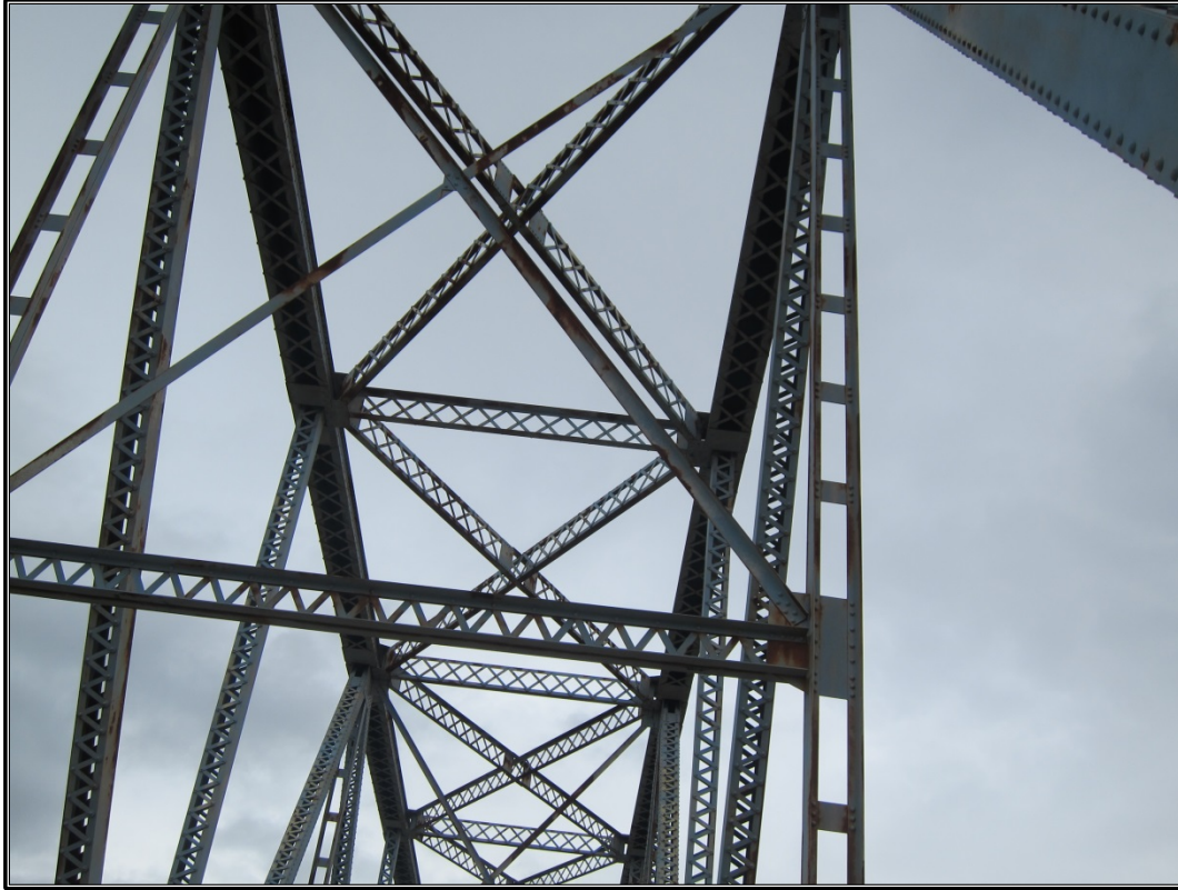
Figure 23. Site 1 (LVS 35): Lattice bracing.
