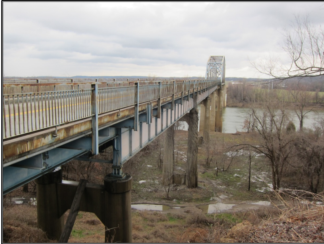
Figure 21. Site 1 (LVS 35): Southern approach span.
