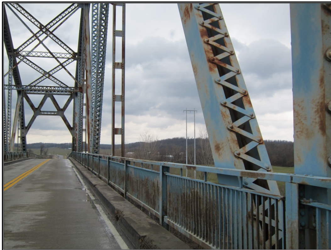
Figure 22. Site 1 (LVS 35): Detail of lacing bars and rivets.
