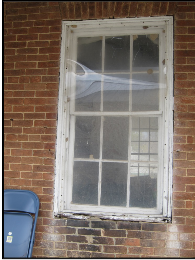
Figure27. Site 4 (LVS 1): Window detail.
