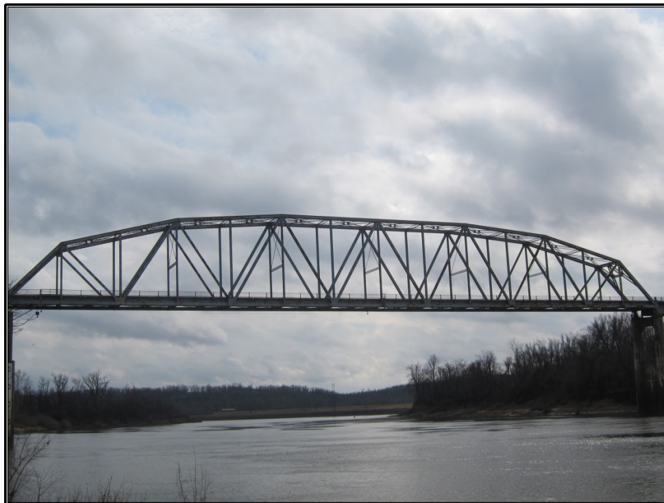
Figure 18. Site 1 (LVS 35): Easterly view of truss span.
