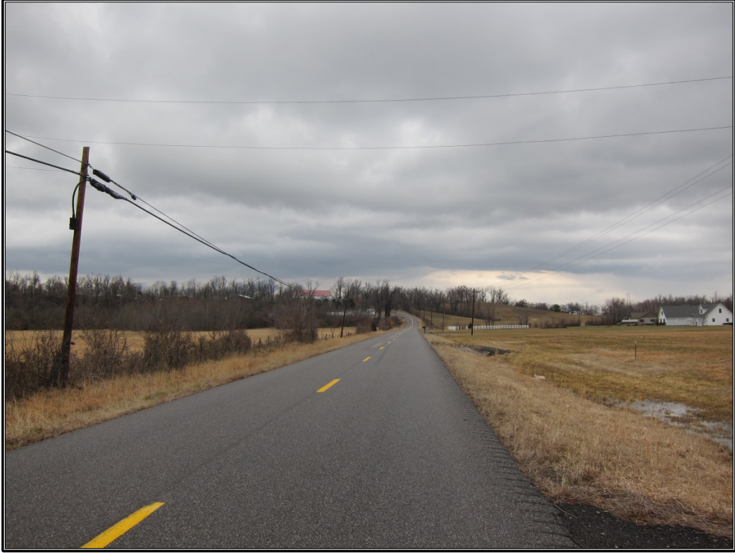
Figure 11. Westerly view of KY 70/Tilne Road.
