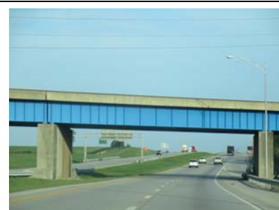
Figure 30. Bridge height is different in different lanes.
