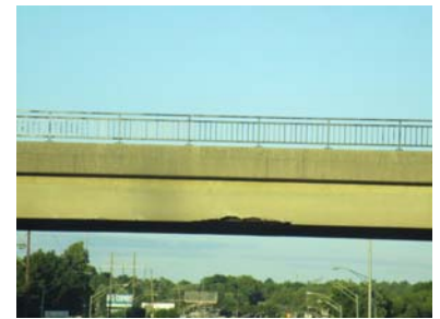
Figure 27. Minor bridge strike near District 7.
