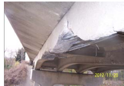
Figure 28. Bridge Strike on Western KY Parkway in 2012 caused major damage.
