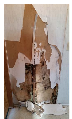
Figure 4. Mold damage to trailer (2014).
