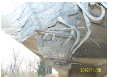
Figure 29. View of bridge Strike in Elizabethtown from underneath.
