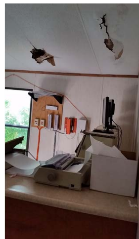
Figure 3. Ceiling caving in because of leakages at Fulton Weigh Station (2014).
