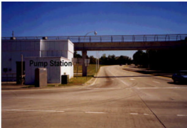
Figure VI- 3. Wilkinson Boulevard Pump Station
