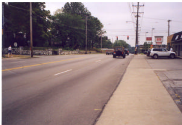
Figure VI- 5. Poor Roadway Edge Delineation
