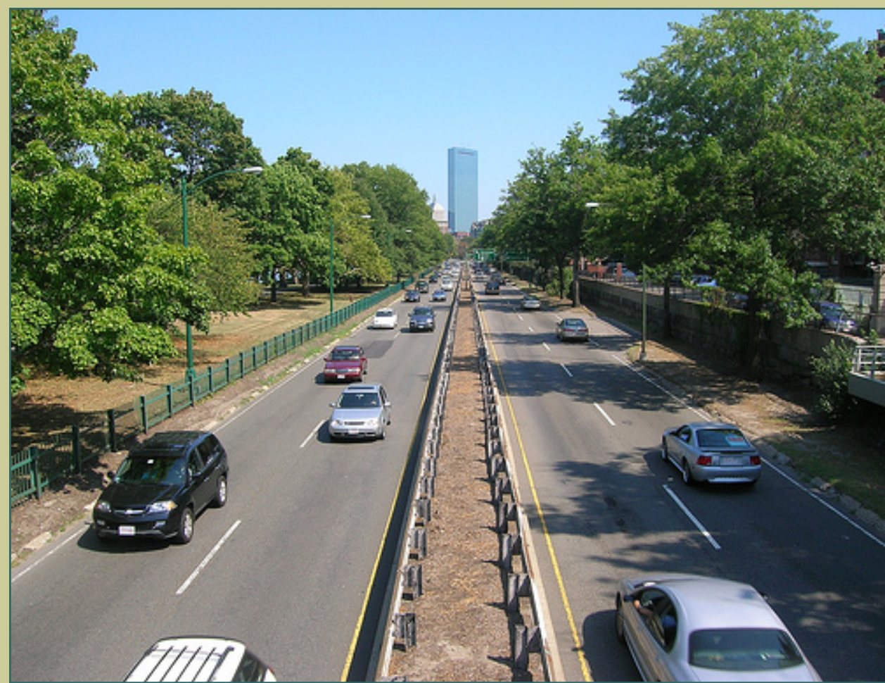
Non-traversable barrier median with no access points
