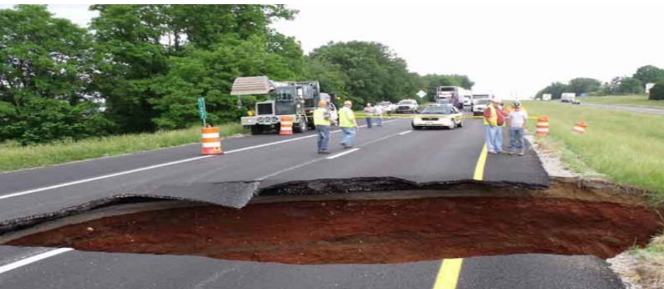
Sinkhole on 1-24 between Nashville and Chattanooga, May 2010
