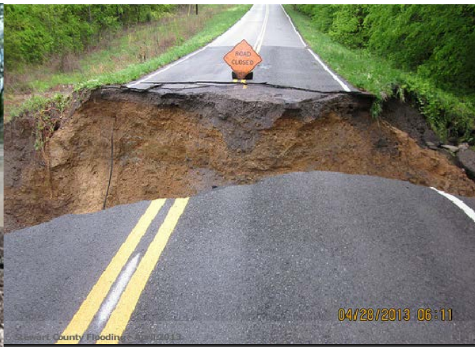
Stewart County Flooding April 2013
