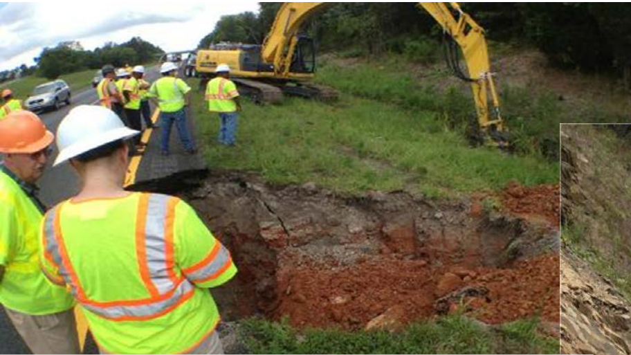
Sinkhole, I-24 Clarksville - August 2013
