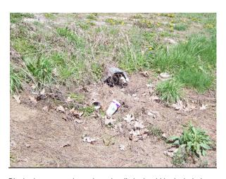
Blocked entrance pipes along the ditch should be included as a ditch obstruction. Circle  $\mathbf{Y}$  if there is any blockage of ditches or entrance pipes along the ditch that inhibit water flow.
